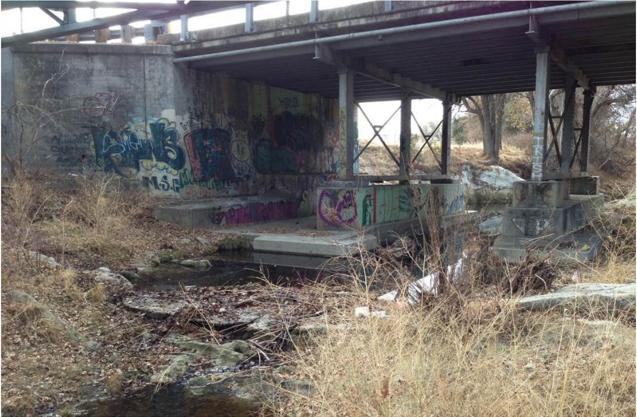
*Figure 11: Concrete check dam downstream of the existing bridge (photo looking upstream)*
