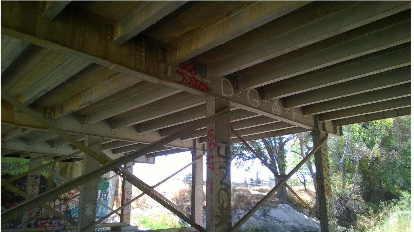
View of steel structure under the bridge. Possible lead based paint a possibility.
