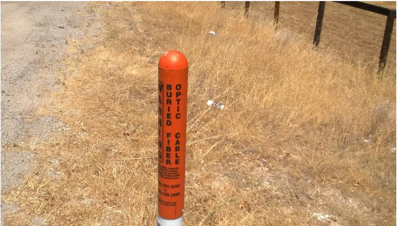
View of fiber optic cable marker along road right-of-way.
