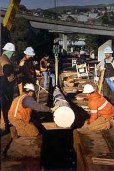
**Gas pipelines being replaced in San Francisco**
