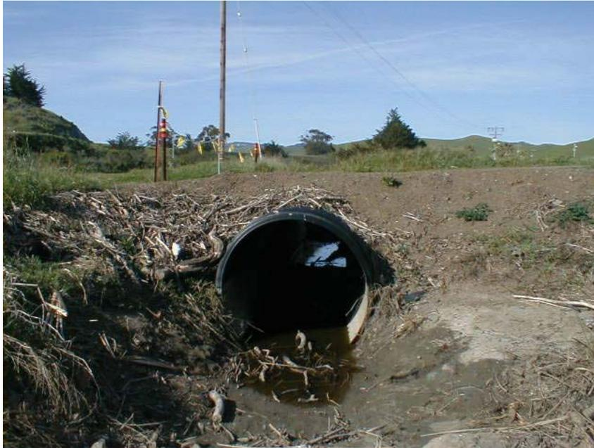
**Photograph 8: 30-inch reinforced concrete pipe culvert at Park Avenue upstream of Third Street drain**
