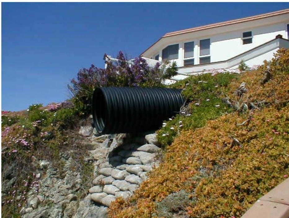
**Photograph 3: Outlet to the 48-inch Caltrans Culvert at Highway 1**
