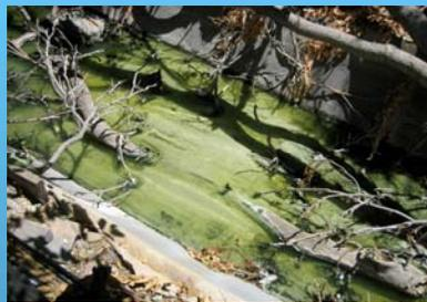
Sulfur precipitates in concrete trench constructed to divert effluent into Salinas River. Water board Required treatment in a leach field.
