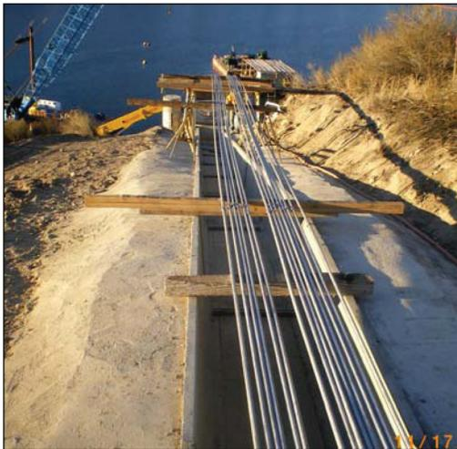
**Figure 3. Preparing for Hydraulic Line Installation**
