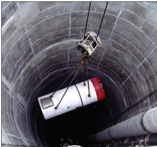
**Figure 8. Placing MTBM in Shaft.**
