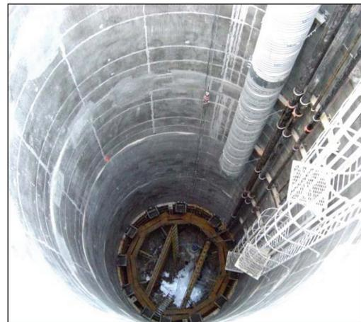
**Figure 6. Pour for Lift 6 - Formwork in Place.**
