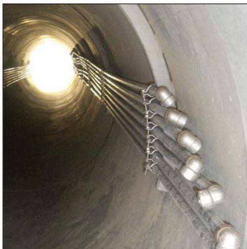
**Figure 4. Hydraulic Lines in Intake Pipe.**
