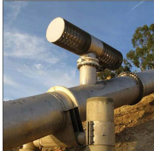
**Figure 9. Fish/Debris Screen.**
