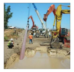
Figure 3. Atascadero Turnout HDD Pullback
