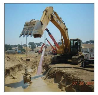
Figure 4. Paso Robles Turnout HDD Pullback.
