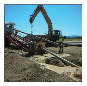
Figure 5. Adding drill stem for MSR HDD.
