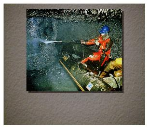
a hot water source and the ability to hold the water in the system during the treatment. Areas that can not be enclosed for thermal treatment can be cleaned with a high-pressure, hot water (140° F) sprayer that will kill the Zebra Mussel instantly and remove them from the surface being cleaned.
