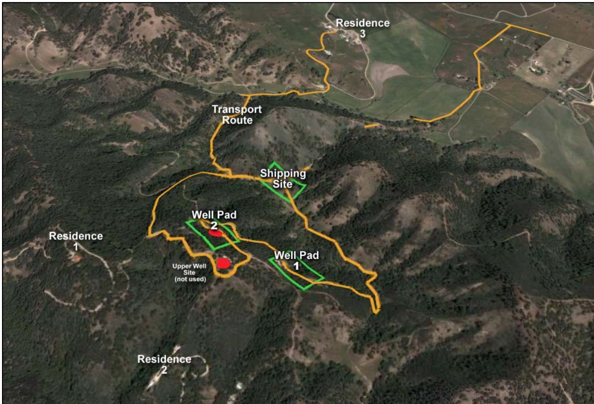
Figure 3: Aerial View of Well Pads and Shipping Site with 3D Topography
