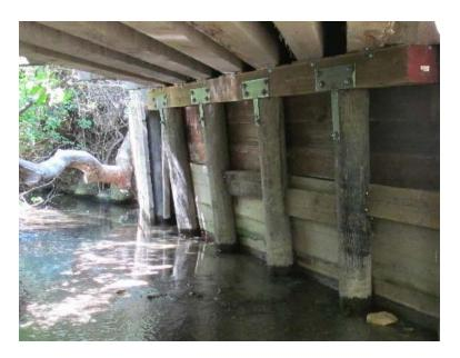
Repaired Timber Cap Beam on Pippin Lane Bridge
