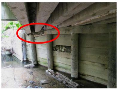
Crushed Timber Cap Beam on Pippin Lane Bridge - Before Repair
