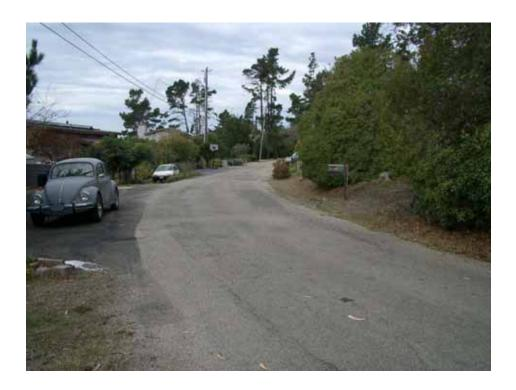
Photograph 6: Homes on McCabe Constructed below Street Grade without Berms or Appropriate Drainage.
