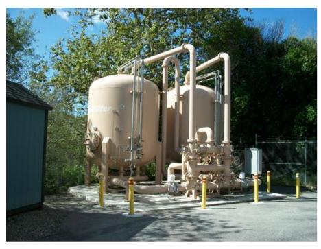
**FIGURE 8: GRANULAR ACTIVATED CARBON FILTERS**
