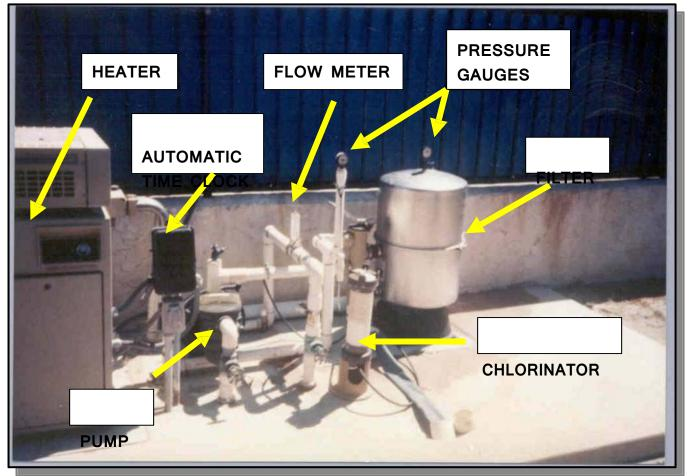
This section provides a brief and general description of the components of a recirculation, filtration and disinfection system of a 30,000 to 40,000 gallon swimming pool. It discusses the different types of filters and disinfection systems that are commonly used in San Luis Obispo County.
