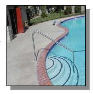
**GUTTERS** are found at large municipal and club pools or older pools built before 1960. Gutters serve two functions: trap debris and scum from the surface of the water and provide a handhold for bathers.
