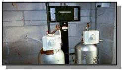
primarily used only to feed carbon dioxide to lower pH. *If you use gas feeders, be* sure that the gas tanks are securely fastened to the wall to prevent them from falling over when accidentally bumped or during an earthquake.
