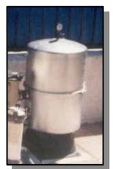
should be disassembled and the filter grids removed, cleaned and inspected for damage. This should be done every 2 to 3 months depending on pool bather load. The local sewer district may also require D.E. separators for these filters, especially if the pool exceeds 2000 square feet. Safer filter media such as Perlite may also be used in D.E. filters. Check with the manufacturer's standards.
