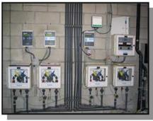
to a computer, the pool's water chemistry can be monitored from off-site locations. These systems provide excellent control of water chemistry by constantly measuring pH and disinfection levels. But routine maintenance of the system can increase initial costs. The
