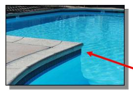
**COPING** around the pool is usually a series of bullnosed stones that slope away from the pool. This helps keep the pool clean by directing water on the deck away from the pool. Coping also functions as a handhold for bathers and must hang over the pool wall at least 1 inch, but not more than 2 inches. It is not to exceed 2  $\frac{1}{2}$  inches in thickness.
