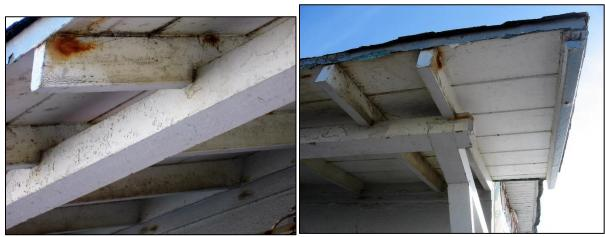
*Figures 47 and 48.* Details of shed-roof extension of roof line on west elevation, sheltering row of windows and doorway. These are not original historic-period features of the Cass Warehouse (compare with Figure 26, above).
