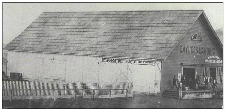
*Figure 25.* This oblique view of the Cass Warehouse shows the original 14 courses of roofing shingles, the mixture of horizontal (front elevation) and vertical (side elevation) wood siding, exterior-mounted sliding barn doors on the side elevation, and the large doorway leading into the warehouse from the loading dock (Source: Cayucos Historical Society).
