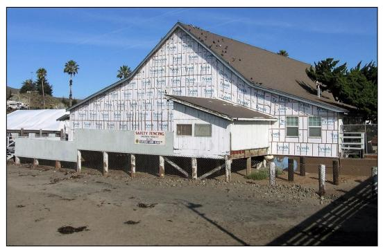
*Figure 44.* Rear view of Cass Warehouse building. The shed-roof addition on the east end of the elevated platform is a modern structure made of older materials.
