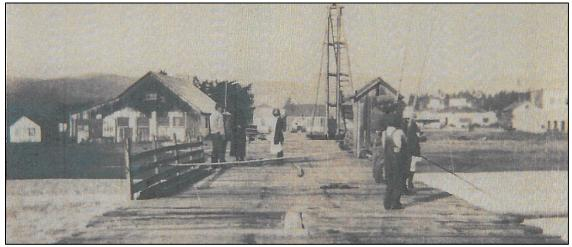
**Figure 23.** In this view from the early 1920s, the warehouse has been relocated to one side of the foot of the pier – its current location. The ancillary storage and warehouse structures have been removed, with only ghosts of paint to show where they had been attached. Original openings in the rear wall of the main warehouse are also visible (Source: Cayucos Historical Society).
