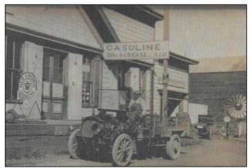
*Figure 24.* An early truck parks outside the warehouse near advertising signs for gasoline and automobile services. Ironically, the rise of trucking helped bring an end to the era of coastwise shipping. The photo provides good documentation of the materials and features used on the front elevation of the warehouse, including doors, windows, horizontal wood siding, roof overhang, and loading dock (Source: Cayucos Historical Society).
