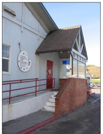
*Figure 43.* Modern signage, access ramp, stairs, railings, door, and glass-enclosed portico associated with Cayucos Community Art Gallery portion of Cass Warehouse building. The doorway itself is probably original to the warehouse building (compare with Figure 29, above).
