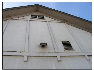
*Figure 42.* Gable end on principal elevation with modern applied wood grid decoration. The broad eaves are original to the historic warehouse structure (compare with Figure 29 above).
