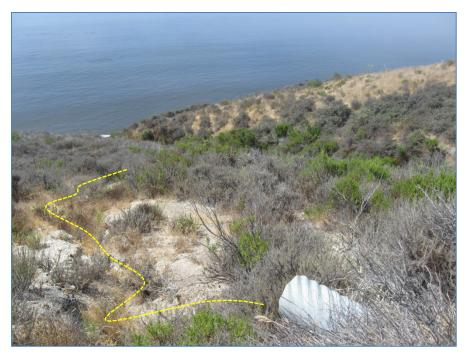
Photo 7. Erosional feature downslope of Culvert 3, facing southwest. The gully is west of this erosional feature.
