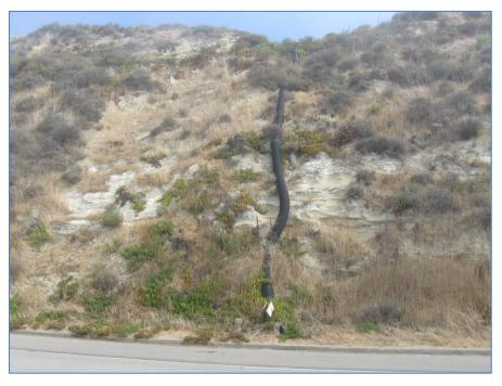
Photo 18. Overflow culvert (Culvert 5) from Culvert Collection Basin 2 conveying flow down the coastal bluff and onto the shoulder of Avila Beach Drive, facing north.
