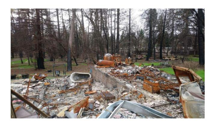
You can see the stucco plaster, which has not burned (after all, it is cement), while all the wooden parts of the house (OSB, 2x4 boards) have burned down completely.
