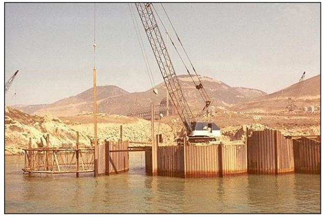
Figure 2-22. Photo from Original Intake Structure Cofferdam Construction
