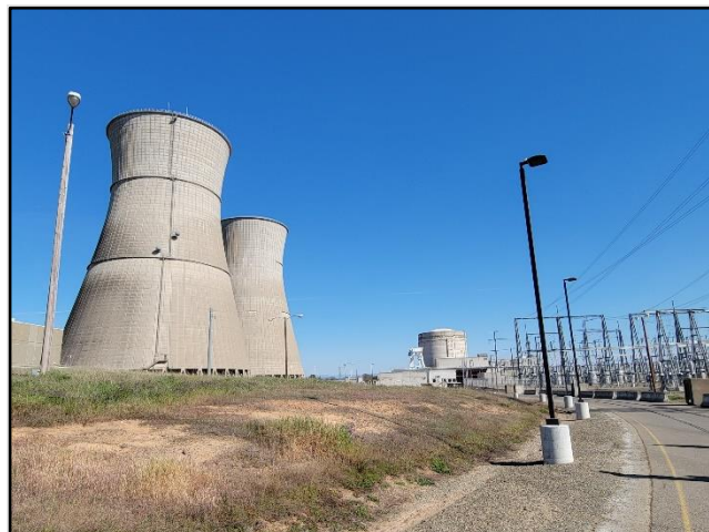
Figure 5-5. Rancho Seco Nuclear Generation Station SAFSTOR Condition
