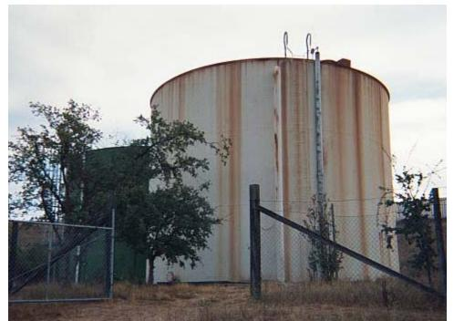
Figure 4 – Existing CSA 23 Welded Steel Tank
