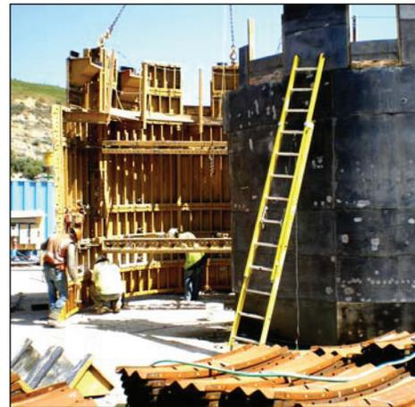
**Figure 5. Preparing Shaft Concrete Form.**
