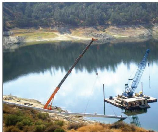
**Figure 10. Placing Intake Pipe**
