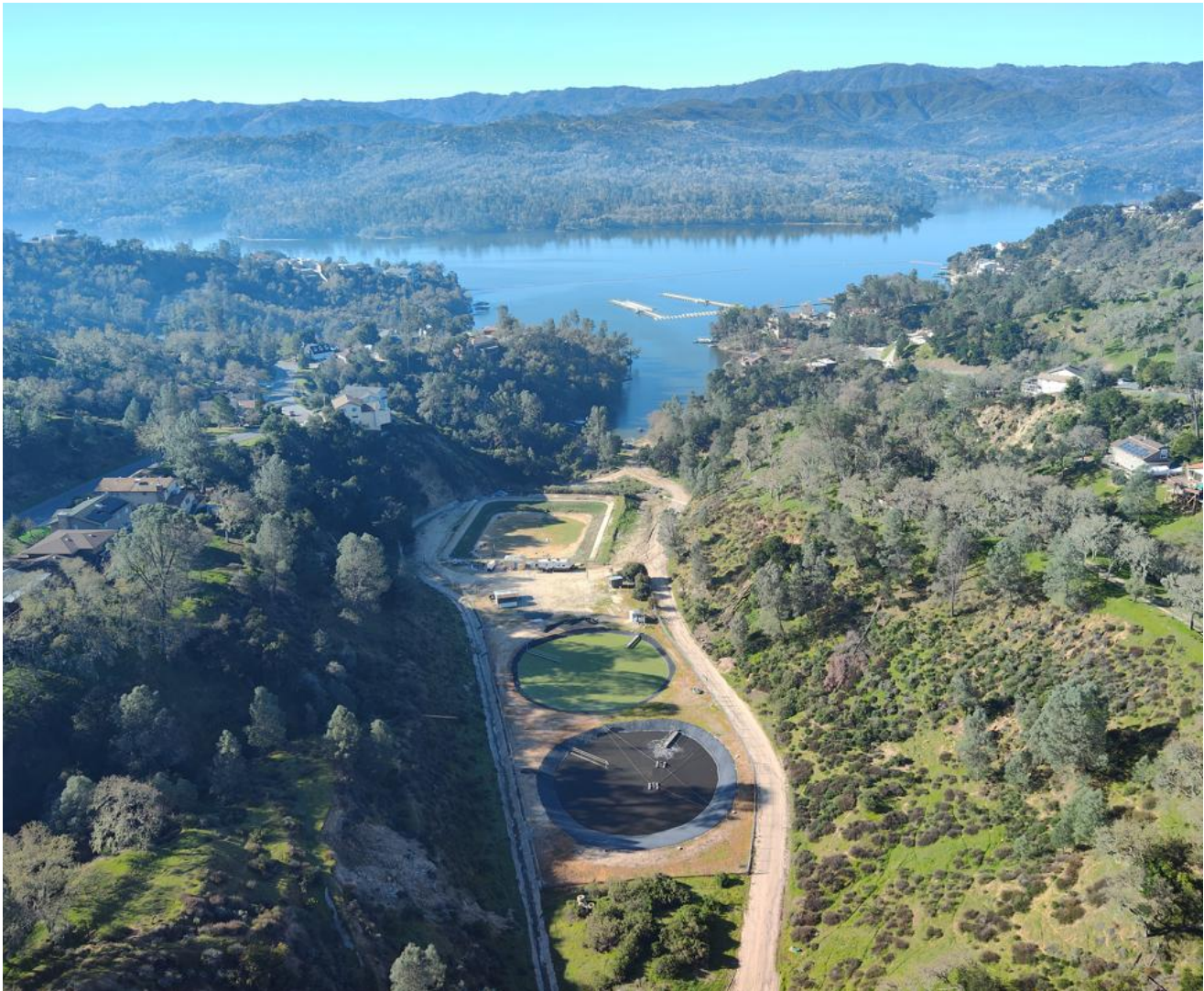
Figure 4: CSA 7A Oak Shores Wastewater Treatment Facility
