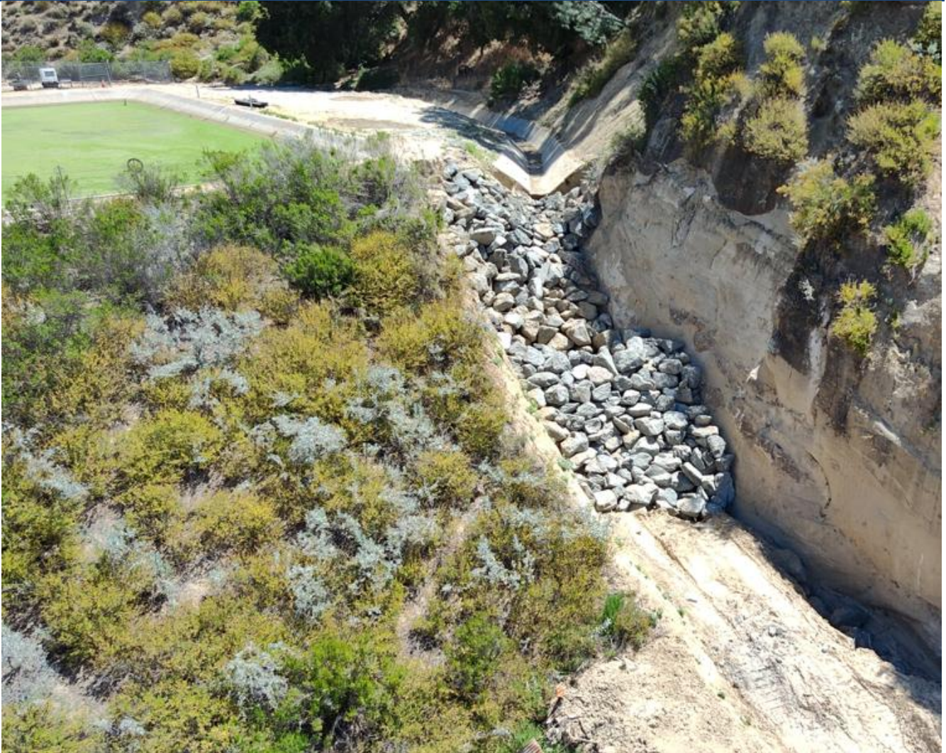
Figure 5: Interim Storm Repair at CSA 7A
