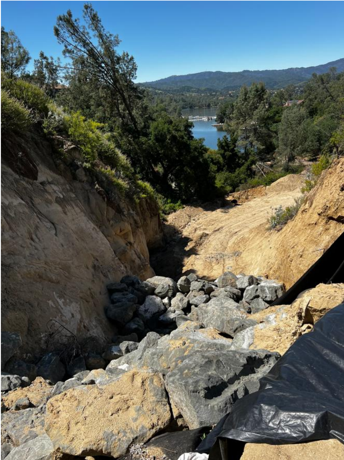
Interim Boulder Stabilization
