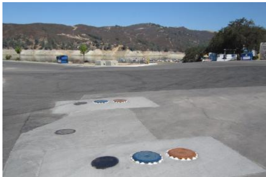
Figure 9: Underground fuel storage tanks loading ports at Lake Nacimiento Resort
