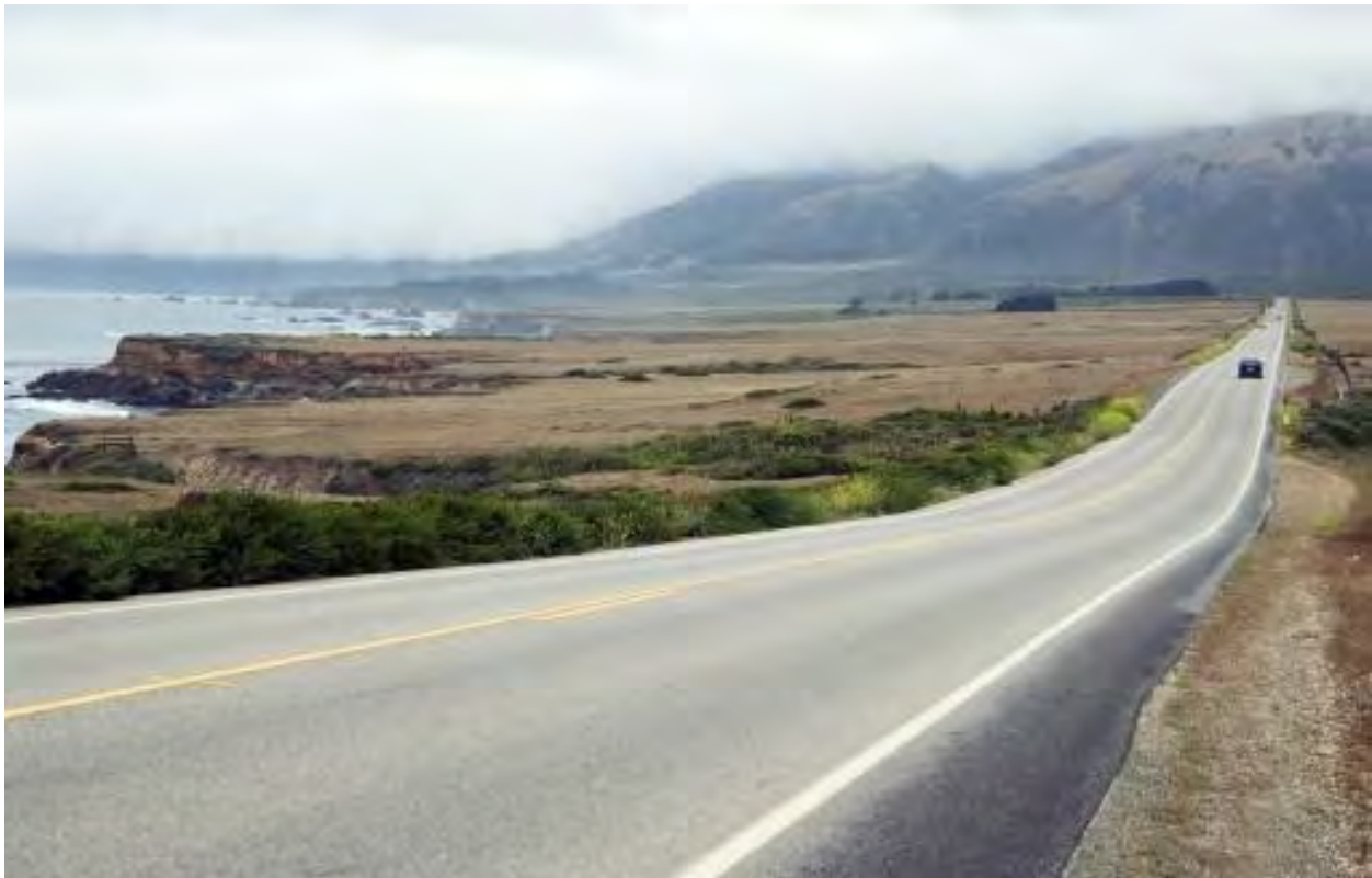
Figure 5-44 Low-lying Portions of Highway 1 in San Luis Obispo County
