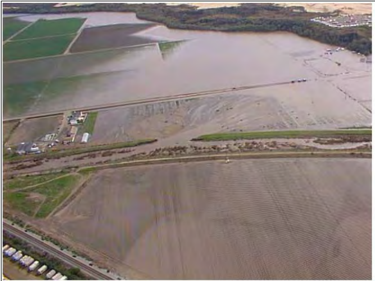
Figure 5-83 Arroyo Grande Levee Failure Event, March 2001 (Looking South)
