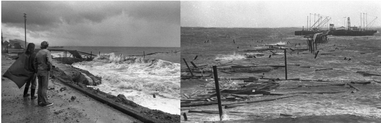
Figure 5-38 Union Oil Pier in Avila Beach Collapses Following Severe 1983 Storm
