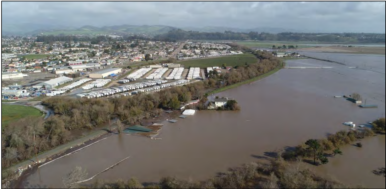
Figure 5-82 South Levee Breach Impacts from the 2023 Arroyo Grande Creek Flooding
