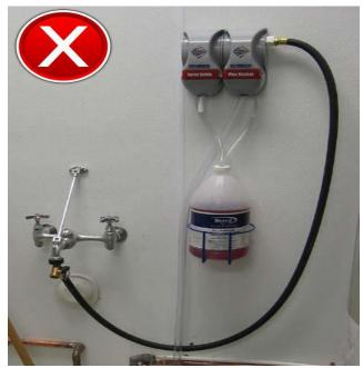
3. Chemical dispenser mounted above AVB; Y-valve attached; hose end below overflow rim of mop sink creating indirect cross-connection.
