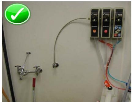
2. Pressure Relief Connection conforming to IAPMO PS-104-2019, downstream of the AVB. Chemical dispenser must still be mounted at least six inches below the AVB.
