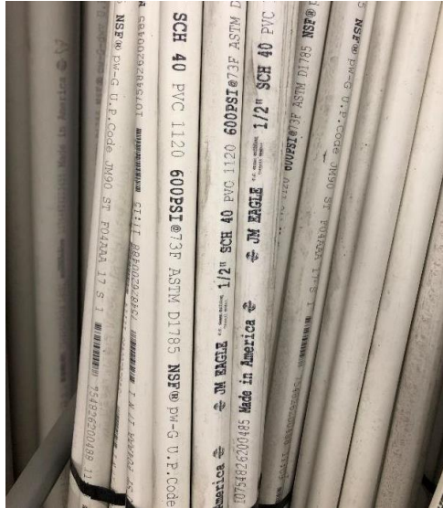
Potable white PVC line with NSF label
