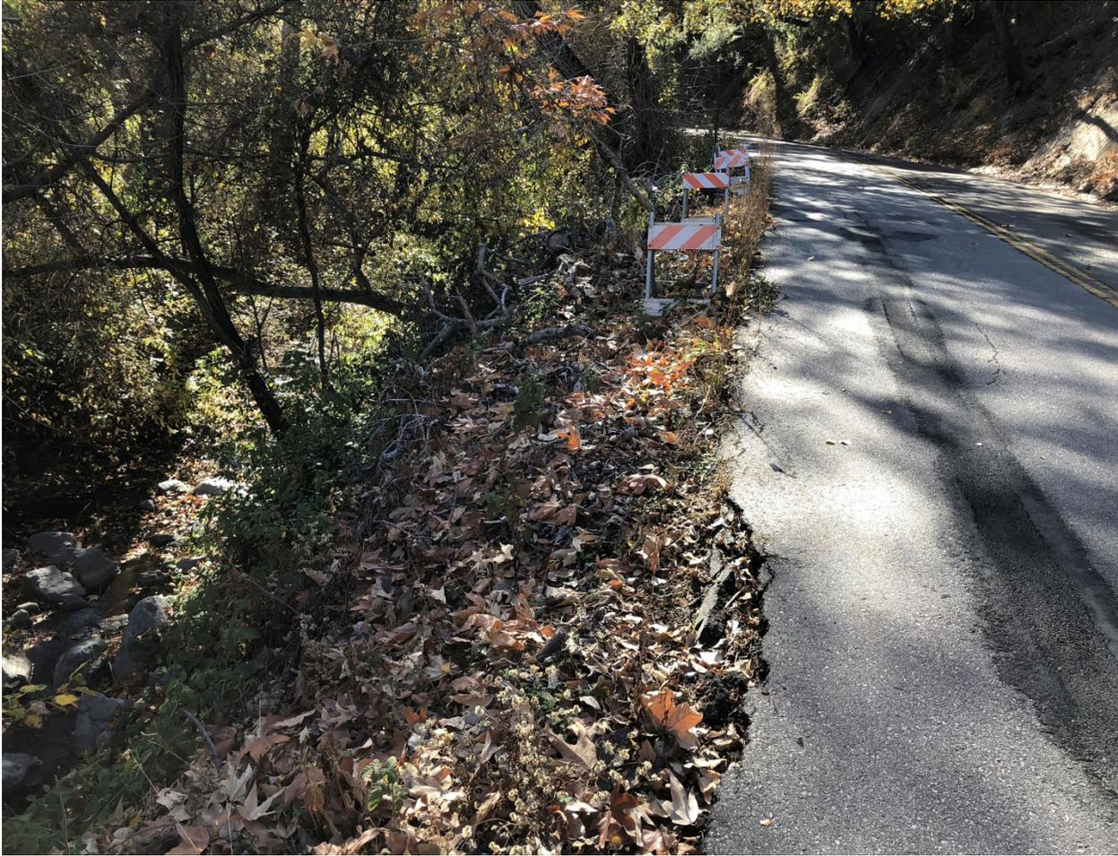
**Figure 4: Eroded Roadway Shoulder on See Canyon Road**
