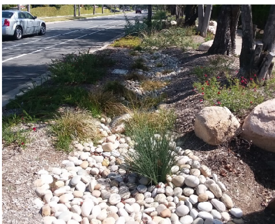
Examples of parkway/LID and curb cuts applications allowing for water infiltration.
