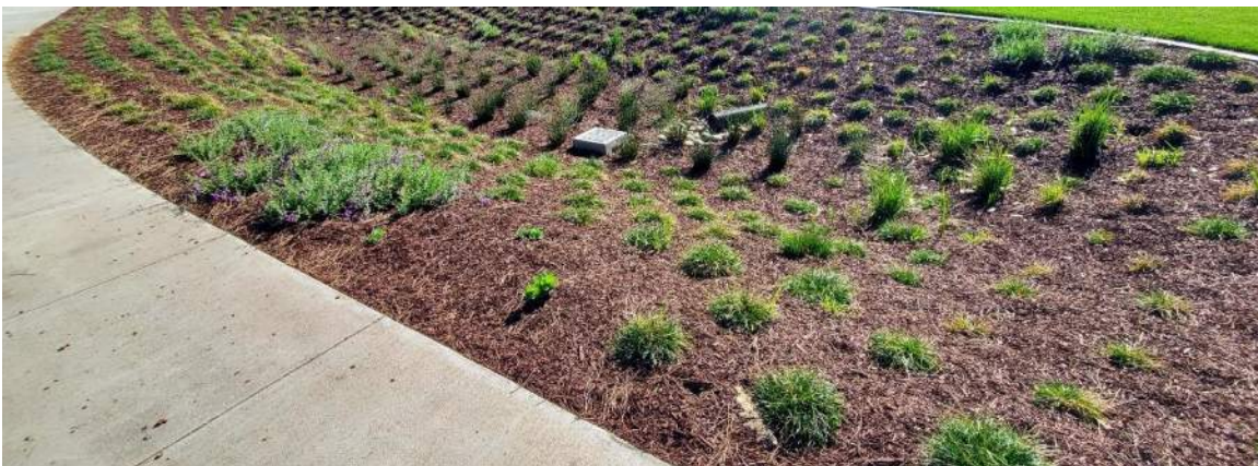
Example of stormwater basin.
