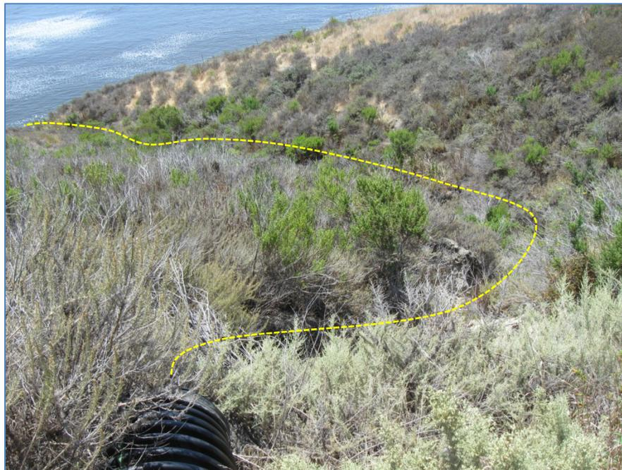
**Photo 4.** Erosion feature downslope of Culvert 2 where a gully has been created, facing southwest.
