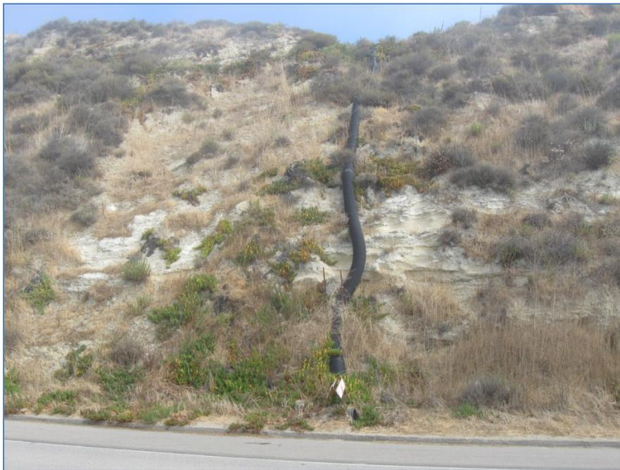
**Photo 18.** Overflow culvert (Culvert 5) from Culvert Collection Basin 2 conveying flow down the coastal bluff and onto the shoulder of Avila Beach Drive, facing north.
