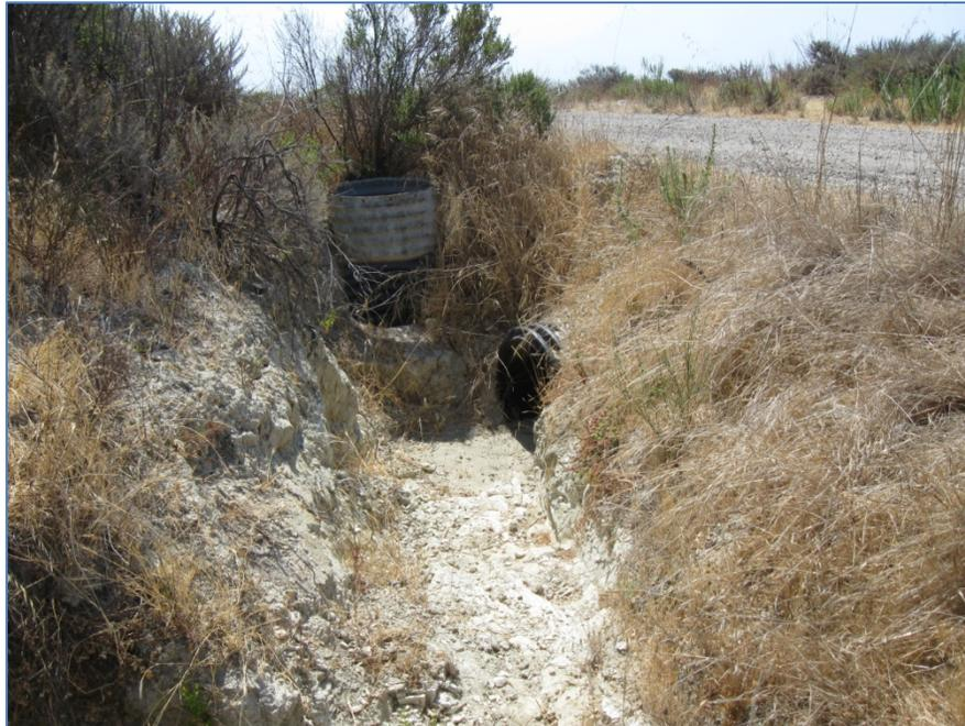
**Photo 3.** Roadside drainage ditch and Culvert Collection Basin1, facing southeast.
