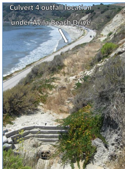
**Photo 16.** Culvert 4 in Culvert Collection Basin 2 that conveys flow down the coastal bluff (under an abandoned access road/erosion control terrace) to a series of standpipes before crossing under Avila Beach Drive and emptying into the ocean, facing west.
