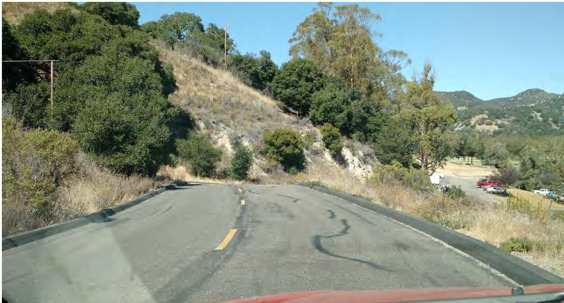
While vehicles exiting the driveway have an ample sight line looking north, the sight distance is only about 120 feet looking south. The vegetation on the southwest corner should be trimmed to ensure vehicles traveling northbound have adequate stopping sight distance approaching the intersection.
