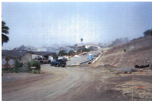
Figure 10: 6-inch Section of Gilbert
