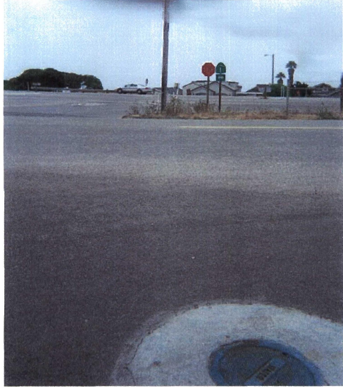
Figure 14: 4-inch Crossing at Highway 1
