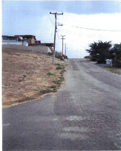
Figure 11: 4-inch on Stuart
