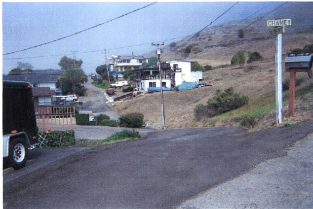
Figure 9: 4-inch Section of Gilbert
