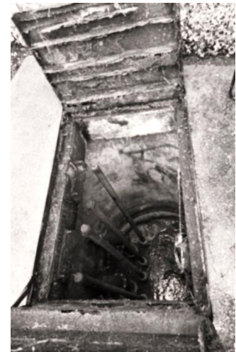
Figure 1: Lift Station 2 w/ Hatch Covers & Pump Guide Rails
