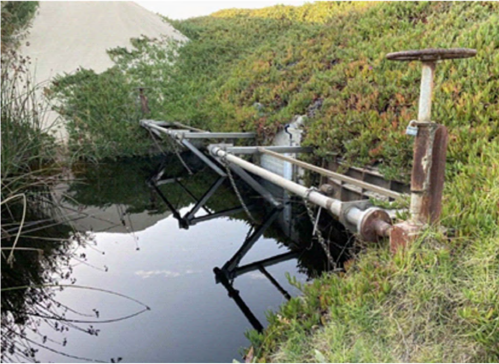
2 PHOTO OF EXISTING TRADITIONAL "FLAP" TIDE GATE TIDE GATES SHOWN TO BE REPLACED WITH VENDOR RECOMMENDED OPTION NTS
