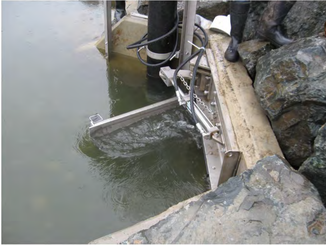
Figure 19. Meadow Creek Lagoon Enhancement Project – 30% Design – Example of a self-regulating side hinge gate.
