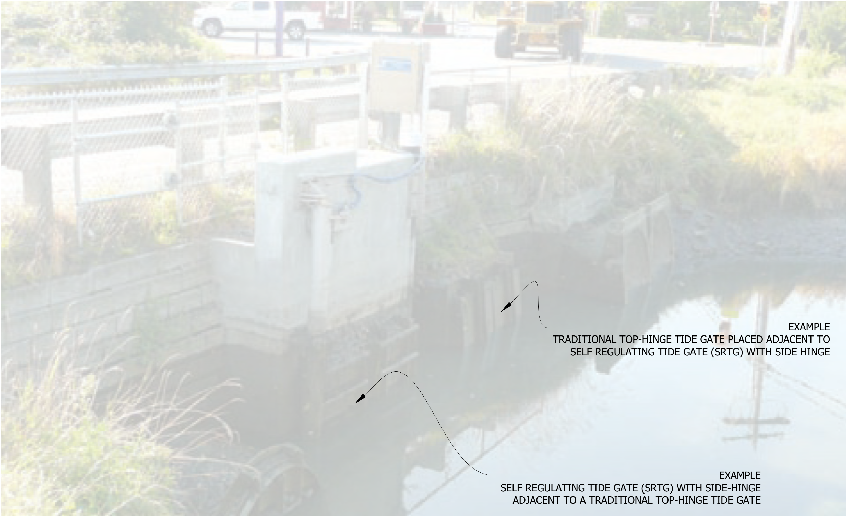
3 PHOTO OF AN EXAMPLE SIDE-HINGE SELF-REGULATING TIDE GATE(S) PAIRED WITH TRADITIONAL TOP-HINGE FLAP GATE(S) EXAMPLE INSTALLATION FOR CONCEPTUAL REFERENCE NTS
