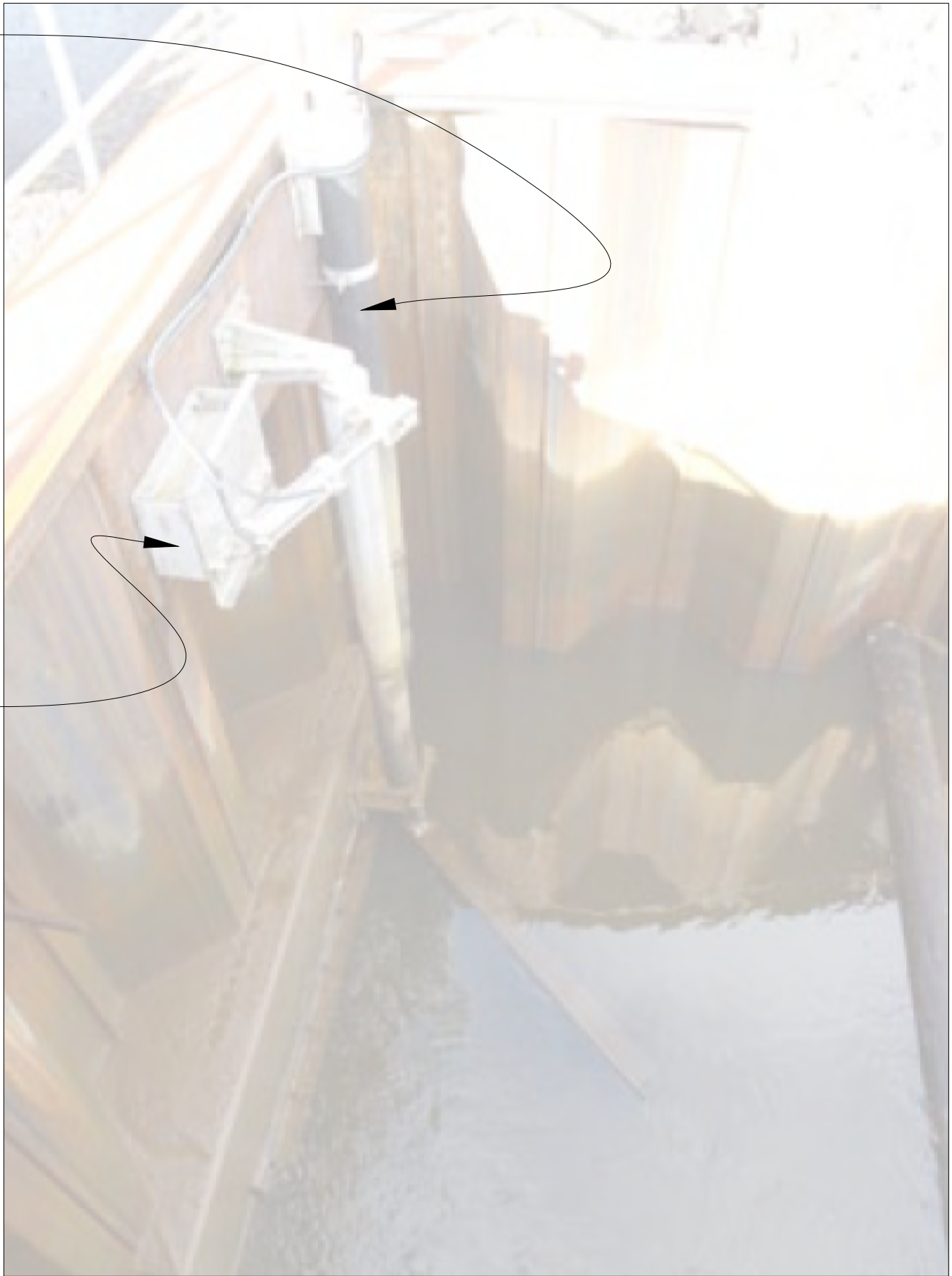
4 PHOTO OF AN EXAMPLE SRT SIDE-HINGE TIDE GATE IN OPERATION EXAMPLE INSTALLATION FOR CONCEPTUAL REFERENCE NTS
