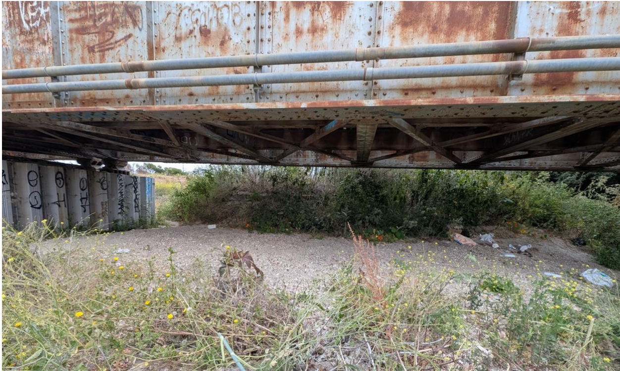
Figure 5: Sediment and Vegetation Blocking the UPRR Bridge Opening, SMZ 7 Looking Downstream (Wallace Group, June 2025)
