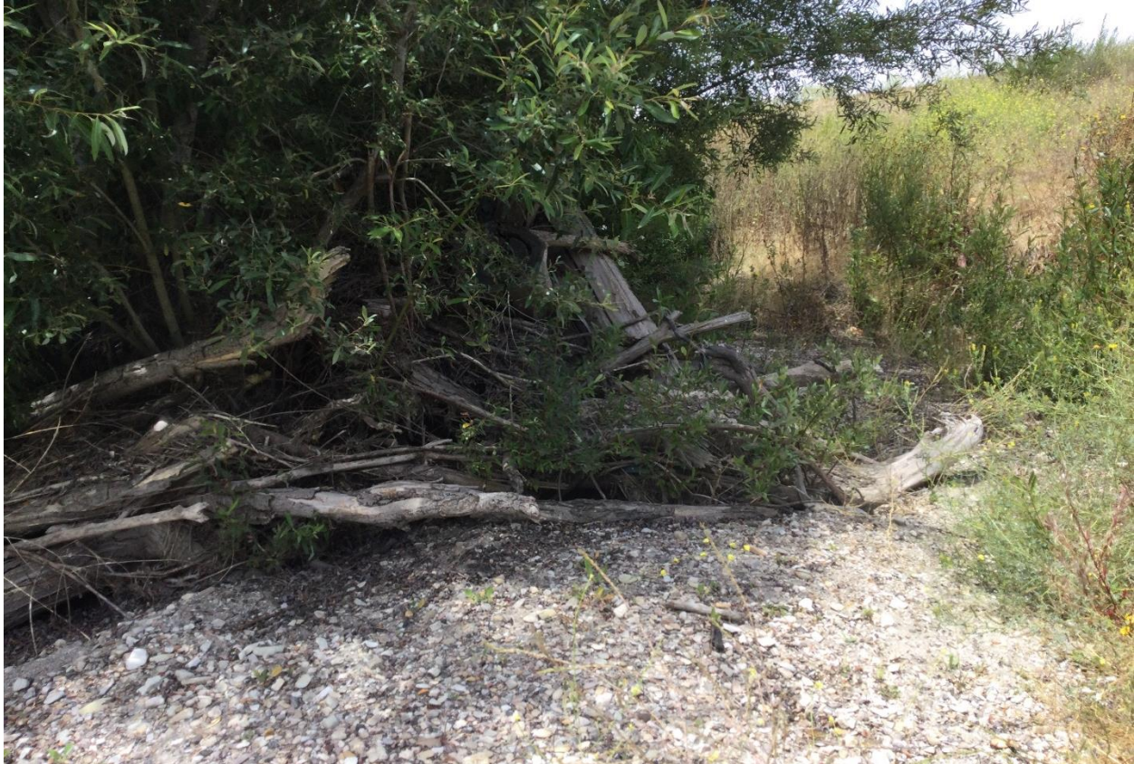
Figure 14: Sediment and Vegetation Buildup at Log Structure 12/13A, Looking Downstream (Wallace Group, June 2025)
