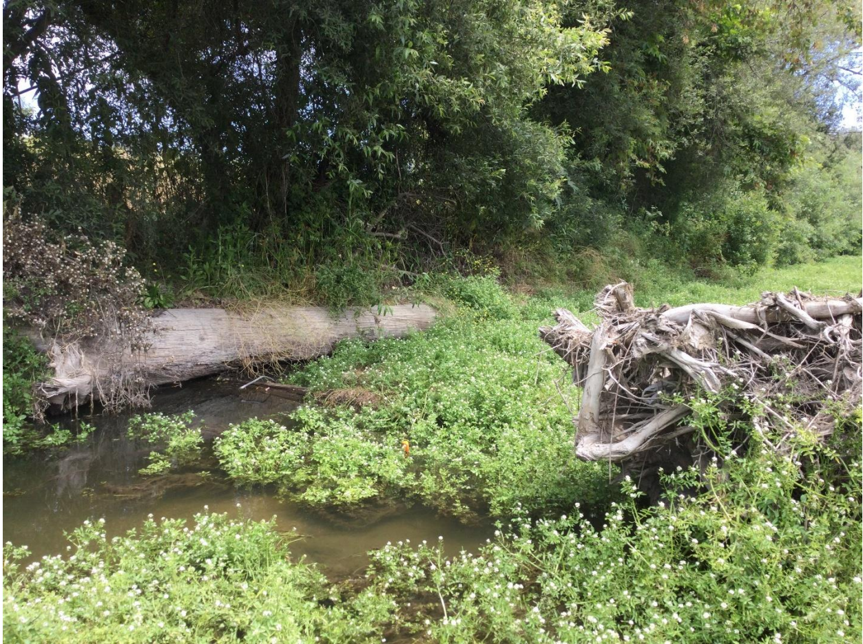
Figure 15: Exposed Log Structure and Root Wads at 14B, Looking Upstream (Wallace Group, June 2025)
