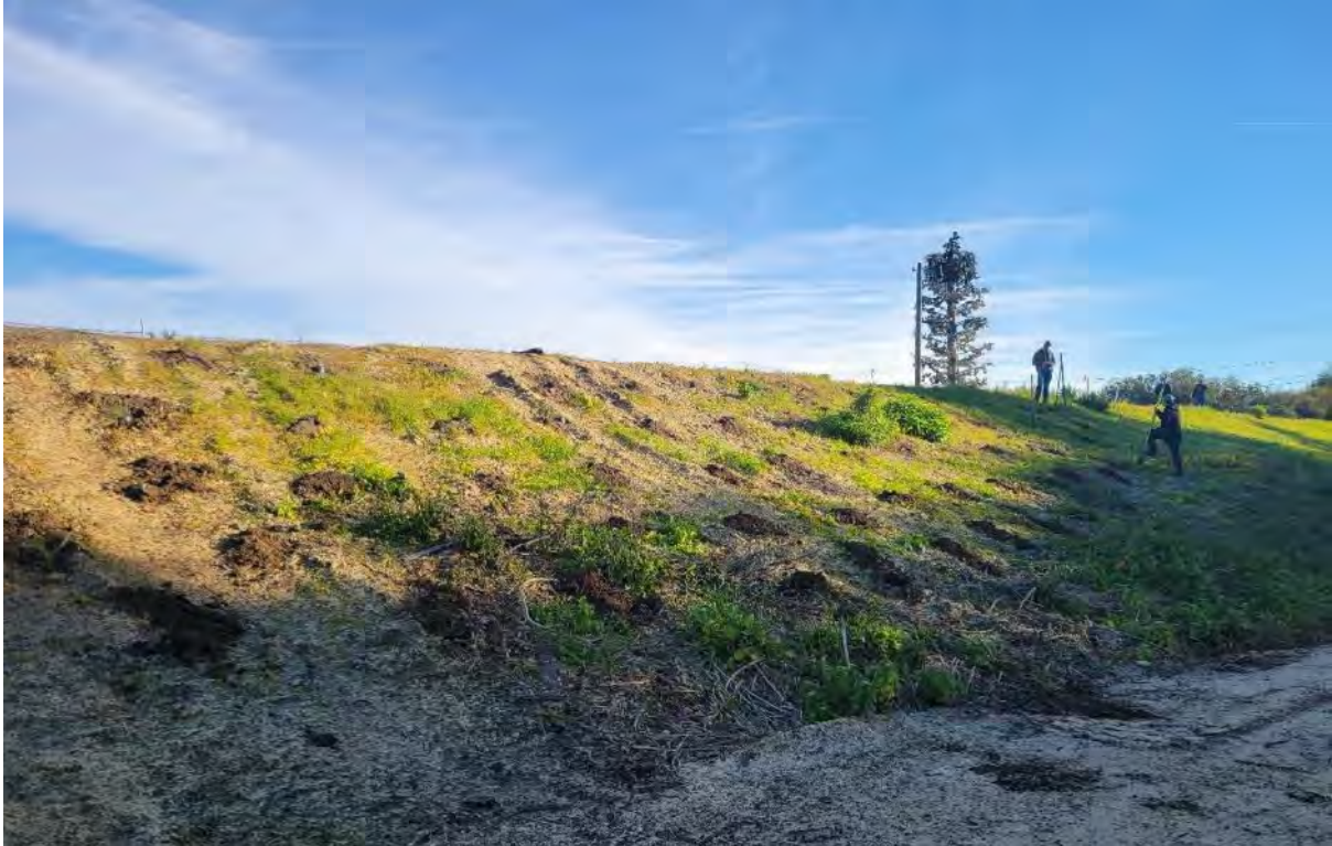
Photograph 17. Planting container plants at SMZ 7. December 2, 2025.
