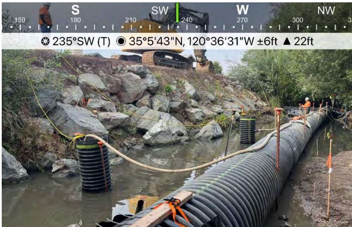
Photograph 12. Looking downstream (southwest) at the Breach Site with diversion pipe and dewatering wells in the foreground. October 21, 2025.
