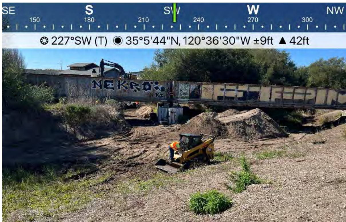
Photograph 10. Sediment removal at SMZ 7. October 16, 2025.
