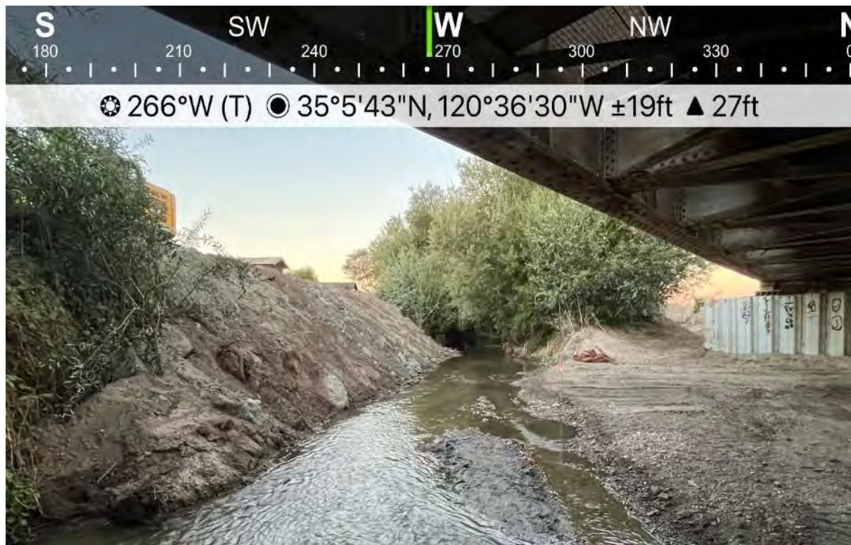
Photograph 16. Looking downstream (west) of Breach Site; levee bank has been stabilized, diversion removed, and streamflow returned to the primary channel. October 28, 2025.
