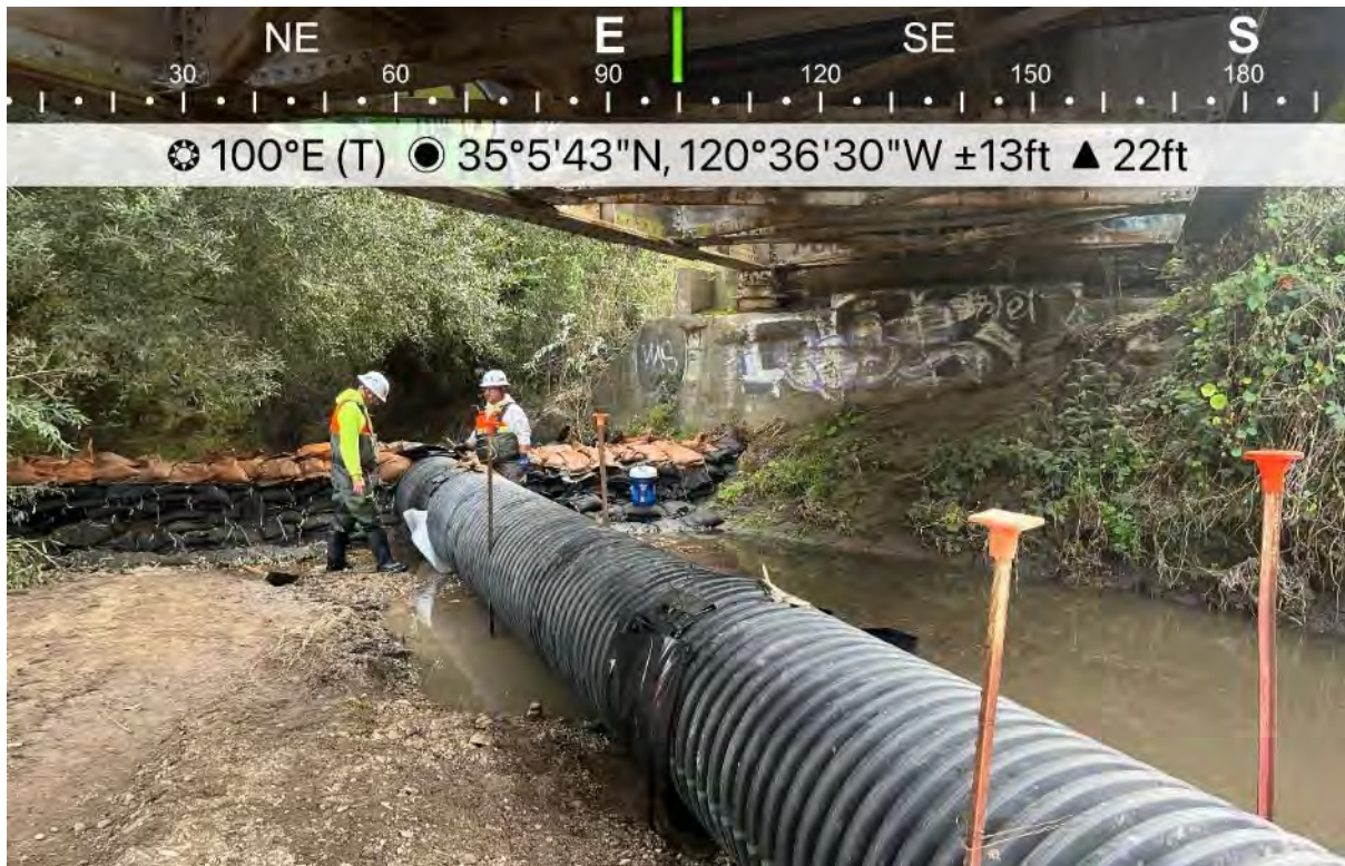
Photograph 11. Looking east at the upstream diversion dam and diversion pipe running under the UPRR Bridge. October 21, 2025.
