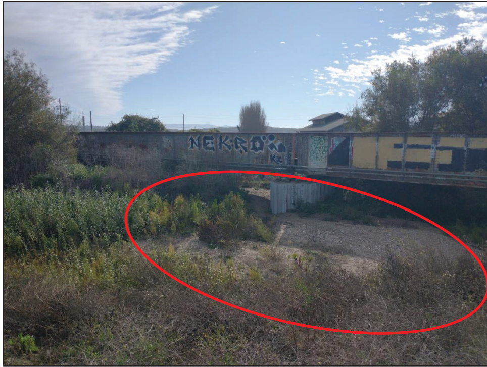
Photo 3. View south of sediment deposition under the Union Pacific Railroad Bridge with SMZ 7 in the foreground and the main channel in the background (December 5, 2024).
