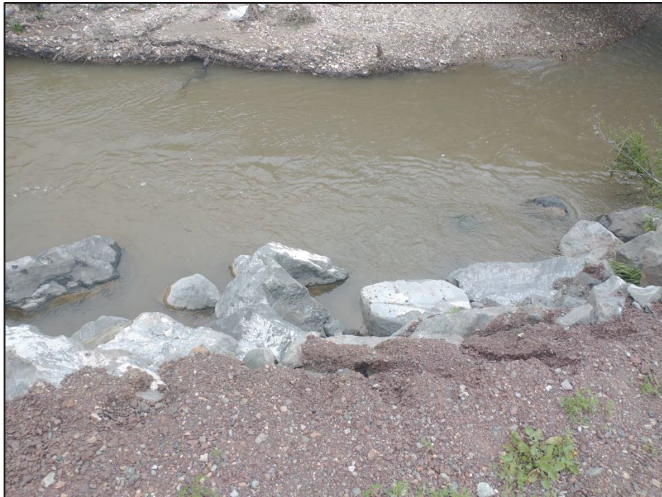
Photo 8. View looking down from the top of the south levee at the breach site repair instability just west of the UPRR (April 3, 2024).
