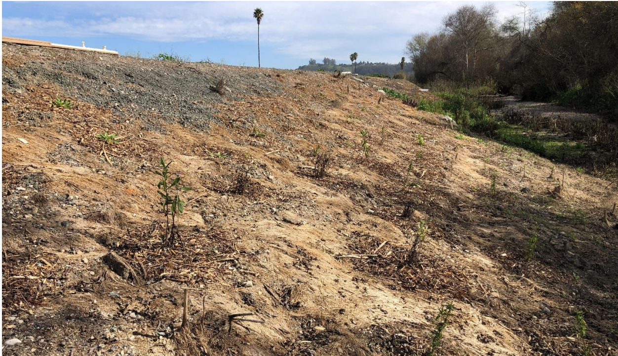
Photo 7. New mitigation container plantings will require maintenance including weed management, addition of arborist wood chips, and potentially supplemental seeding and planting.
