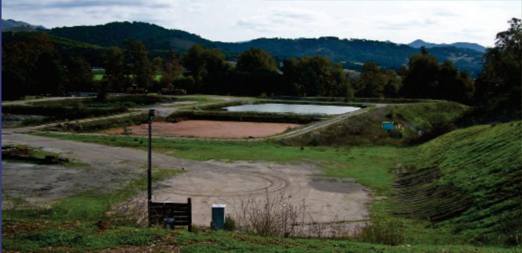
Multiple sludge beds are used to separate materials removed during the various treatment processes.
