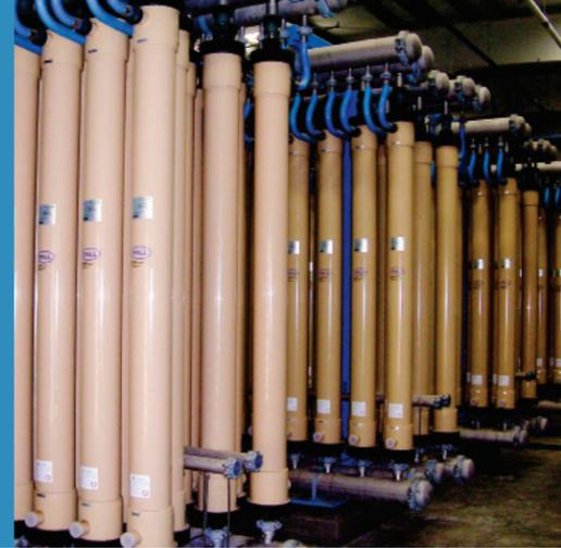
Multiple racks of pressurized membrane filters ensure the removal of all particles and organisms prior to delivery to customers.
