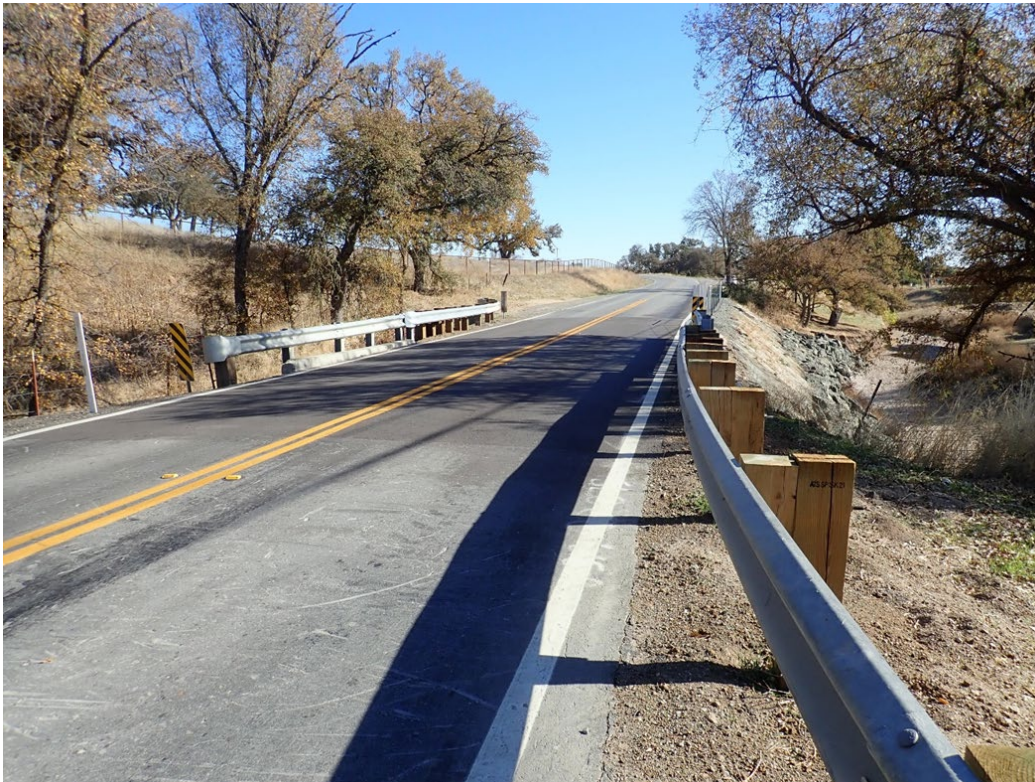
(c) Existing Creston Road Bridge looking east.
