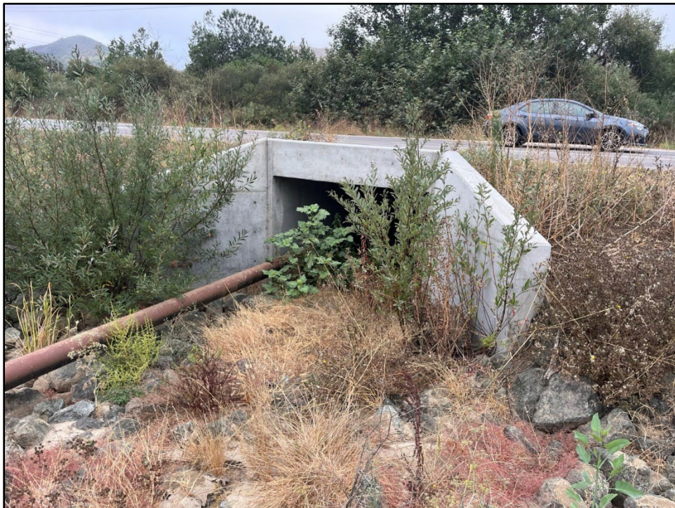
Photo 2. View of the location of Culvert A extension, looking southwest (9-12-2023).
