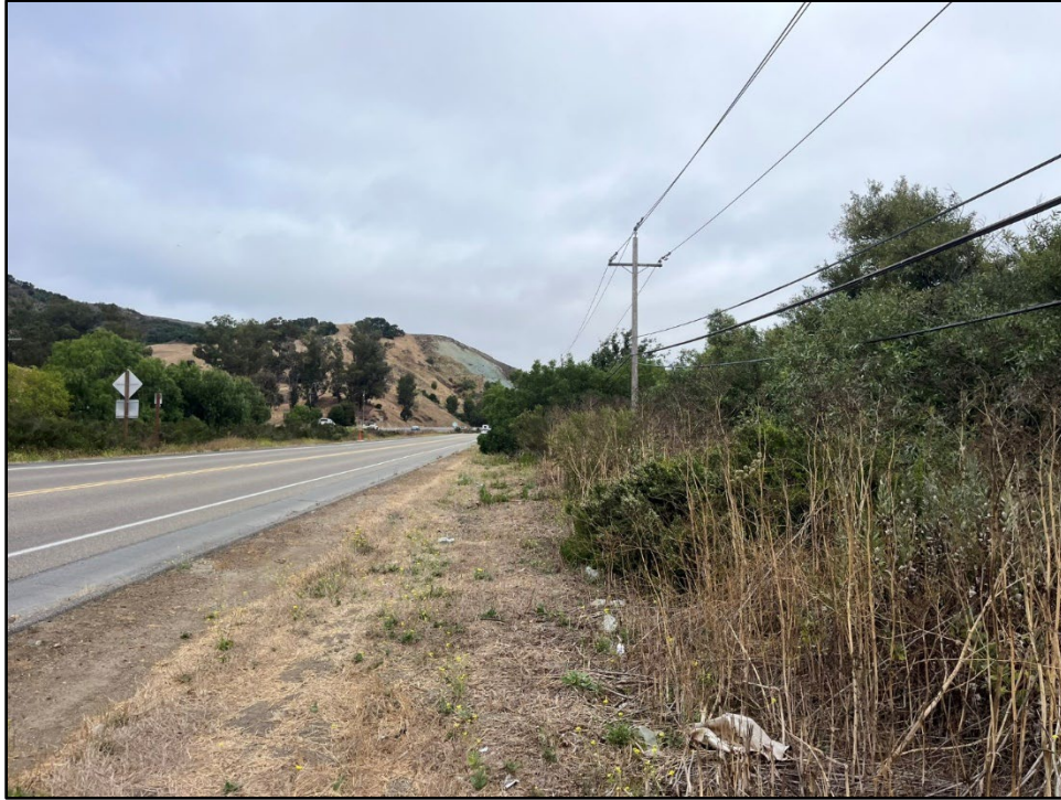
Photo 3. View trail alignment between South Higuera and SLO Creek, looking northwest (9-12-2023).
