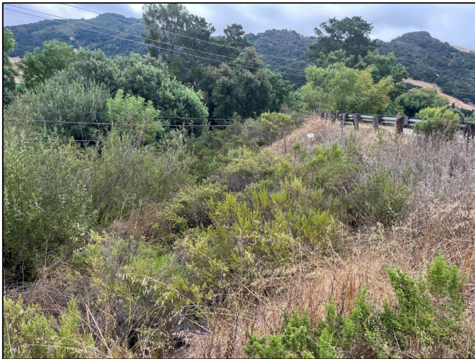
Photo 3. View of the location of the retaining wall north of Cloverridge Lane, looking southeast (9-12-2023).
