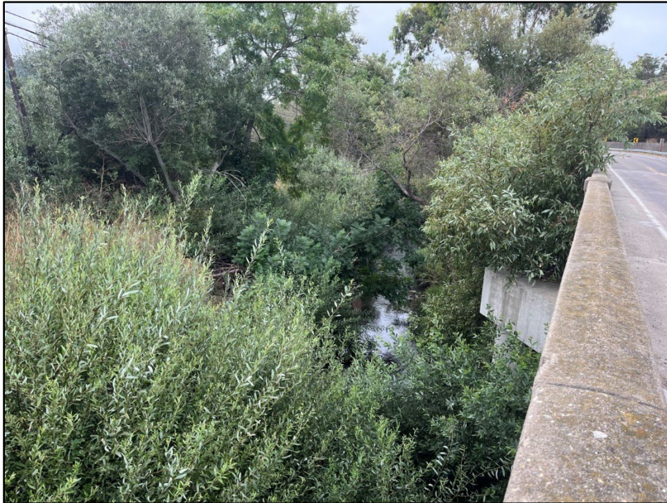
Photo 1. View of SLO Creek downstream of the existing South Higuera Street Bridge where Bridge A will be constructed, looking southwest (9-12-2023).
