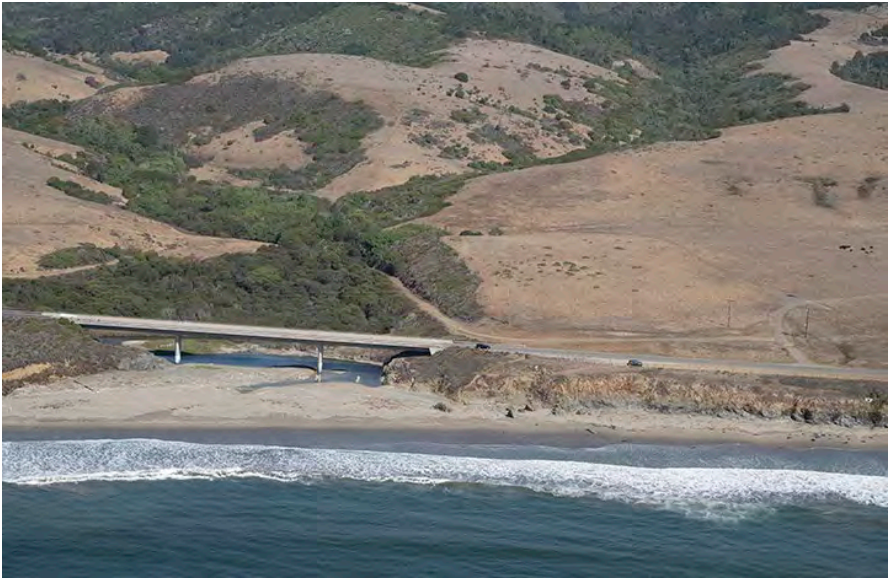
Picture 3. San Simeon - Little Pico Creek Bridge Site
