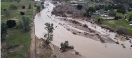
1 Salinas River: 2023 storm events washed out segments of the Nacimiento pipeline; temporary piping is being used during peak season to provide service in the interim.
