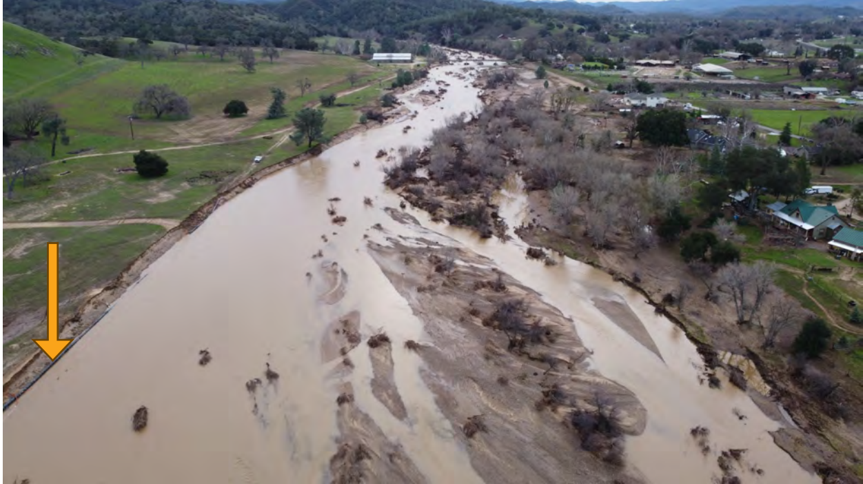
Figure 3.7 Nacimiento Pipeline Damage from 2023 Salinas River High Flows
