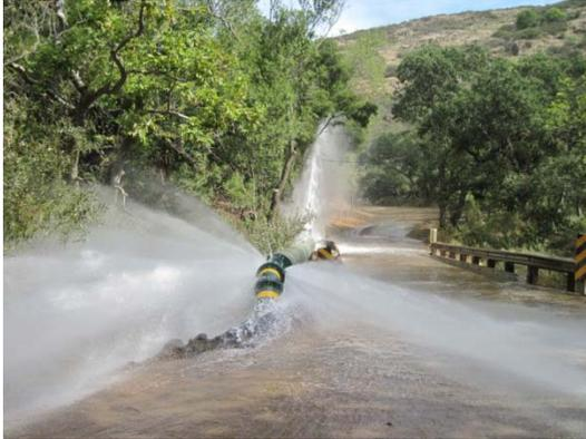
Figure 8 – Pipe Joint Separation at Stenner Creek Bridge
