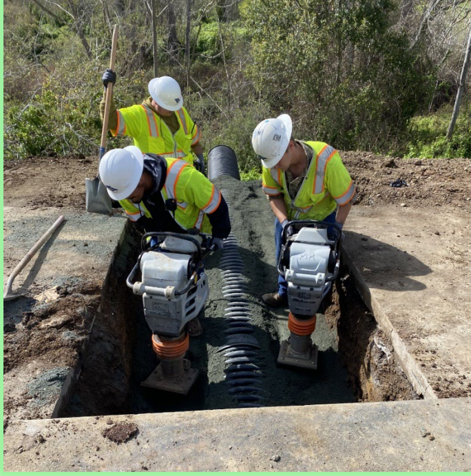
SECTION 3 - CULVERT REPLACEMENT – TORO CREEK RD, MORRO BAY
