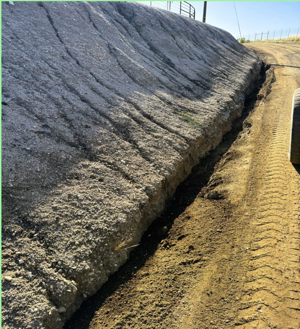
SHOULDER RECONDITIONING – VAQUERO RD, TEMPLETON
