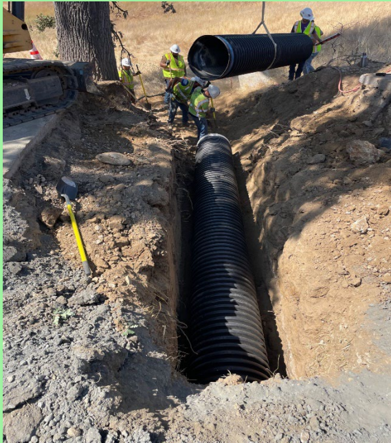
CULVERT REPLACEMENT – CHIMNEY ROCK RD, PASO ROBLES
