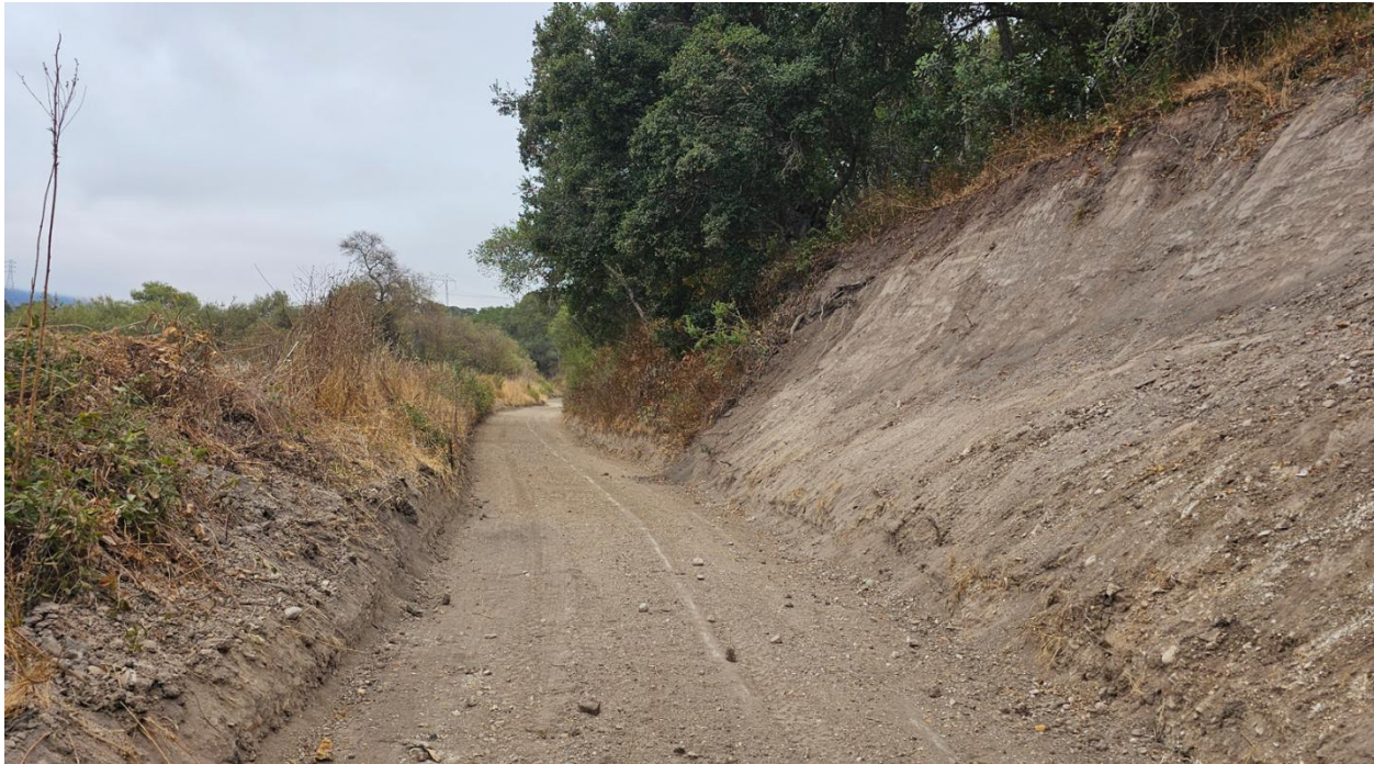
Figure 27: Diversion Channel repair
