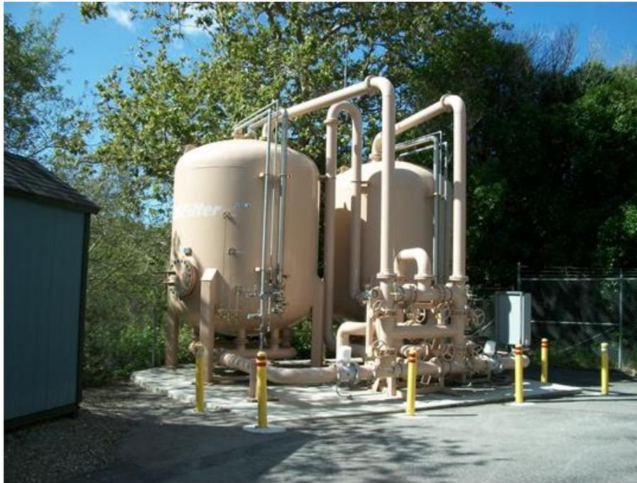
**FIGURE 8: GRANULAR ACTIVATED CARBON FILTERS**
