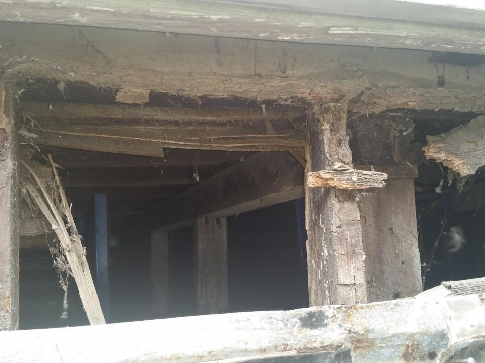
Failed framing connection with rusted/corroded nails
