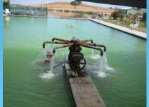
Geothermal well 3458 feet produces 1000 gpm From Monterey Formation
