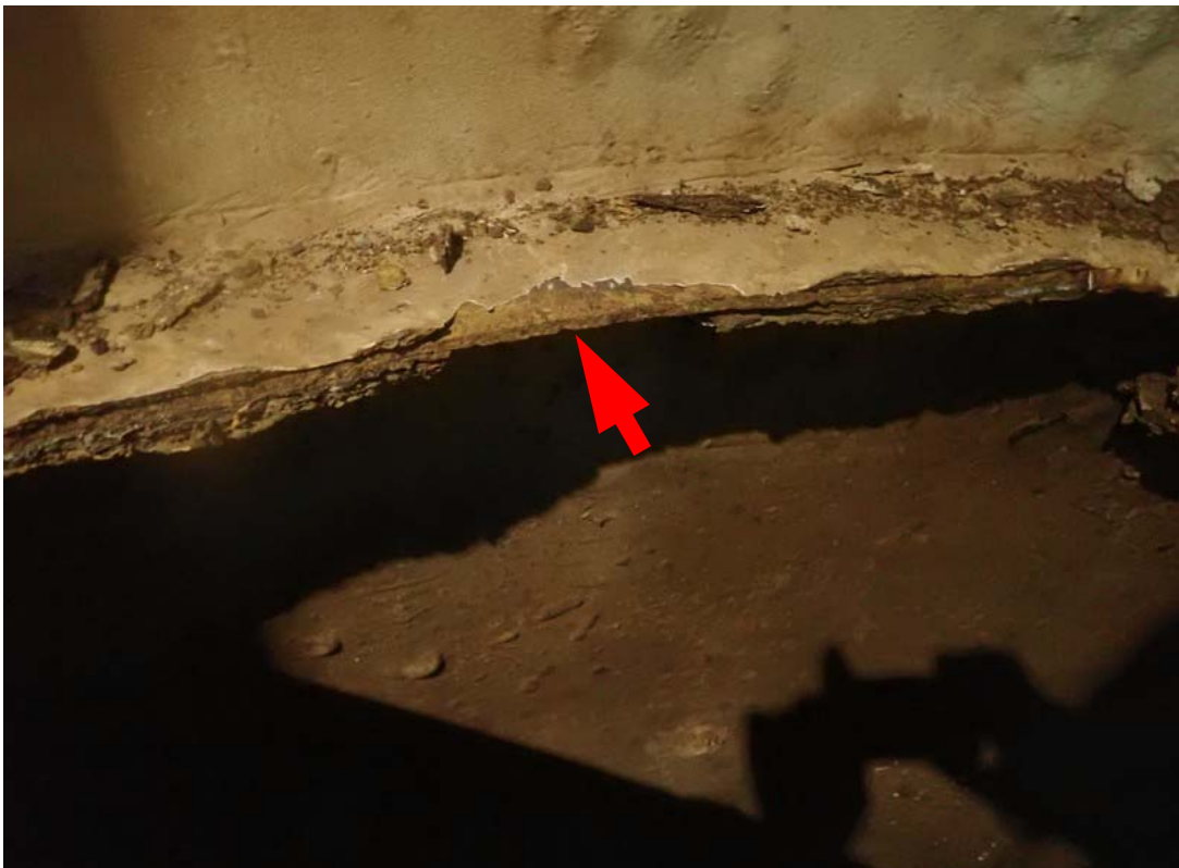
Perimeter "flange" (see top photo for location) after removal of oxides in a sample area (arrow). The corrosion appears the be similar to that found in other areas of the structure.
