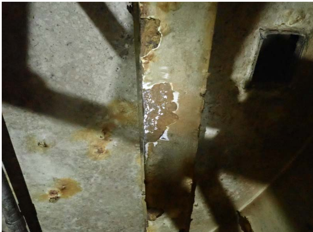
Another view of the bottom side of the hoist beam at a sampled location after removal of loose material.
