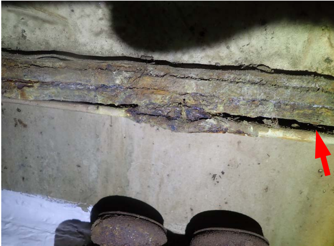
Top flange of hoist beam with inaccessible area above the beam.
