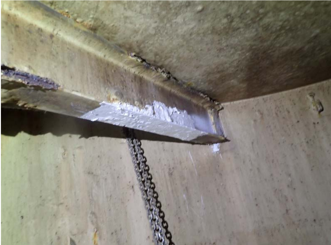
This view shows the spot coating application on a portion of the east beam. The coating was applied over the sample areas where loose materials were removed and the area surrounding the sample areas where loose coating remained.
