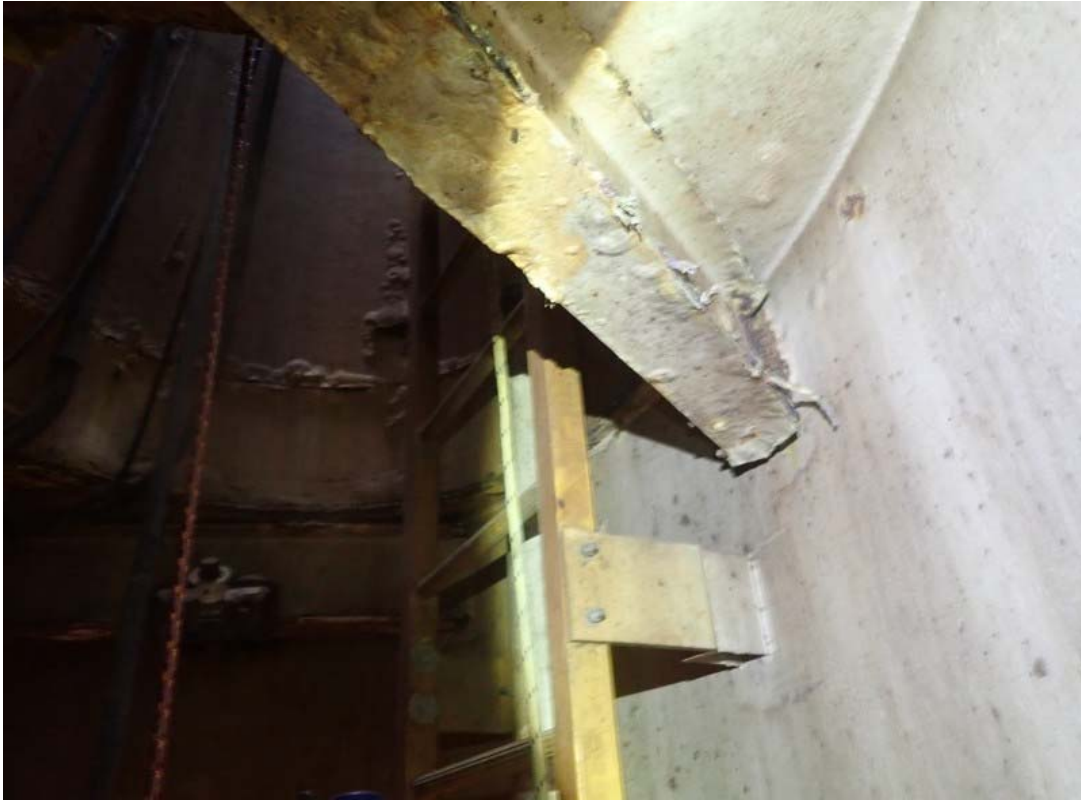
Fiberglass ladder and typical attachment.
