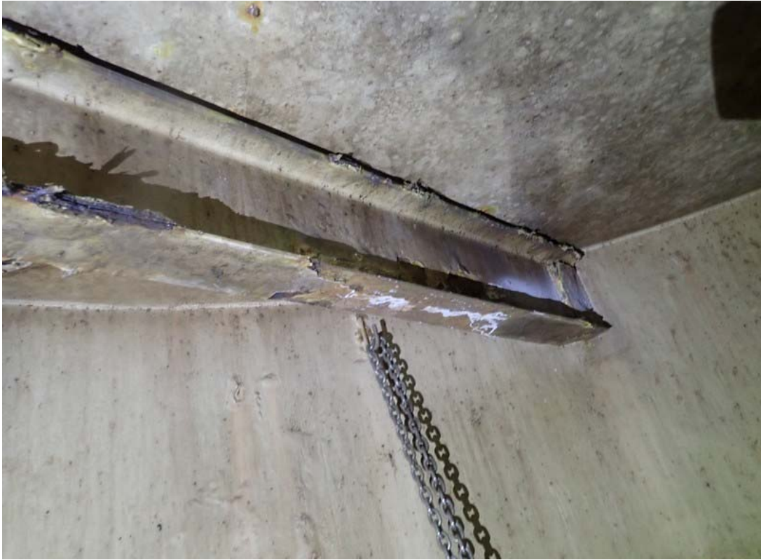
This view shows the south end of the eastern hoist beam (rails). The chain that is visible is part of a pipe support.
