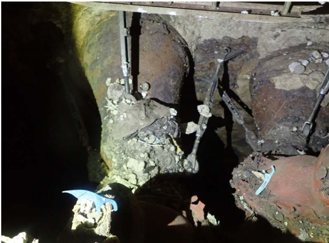
Pipes and hanger turnbuckles under the grating.
