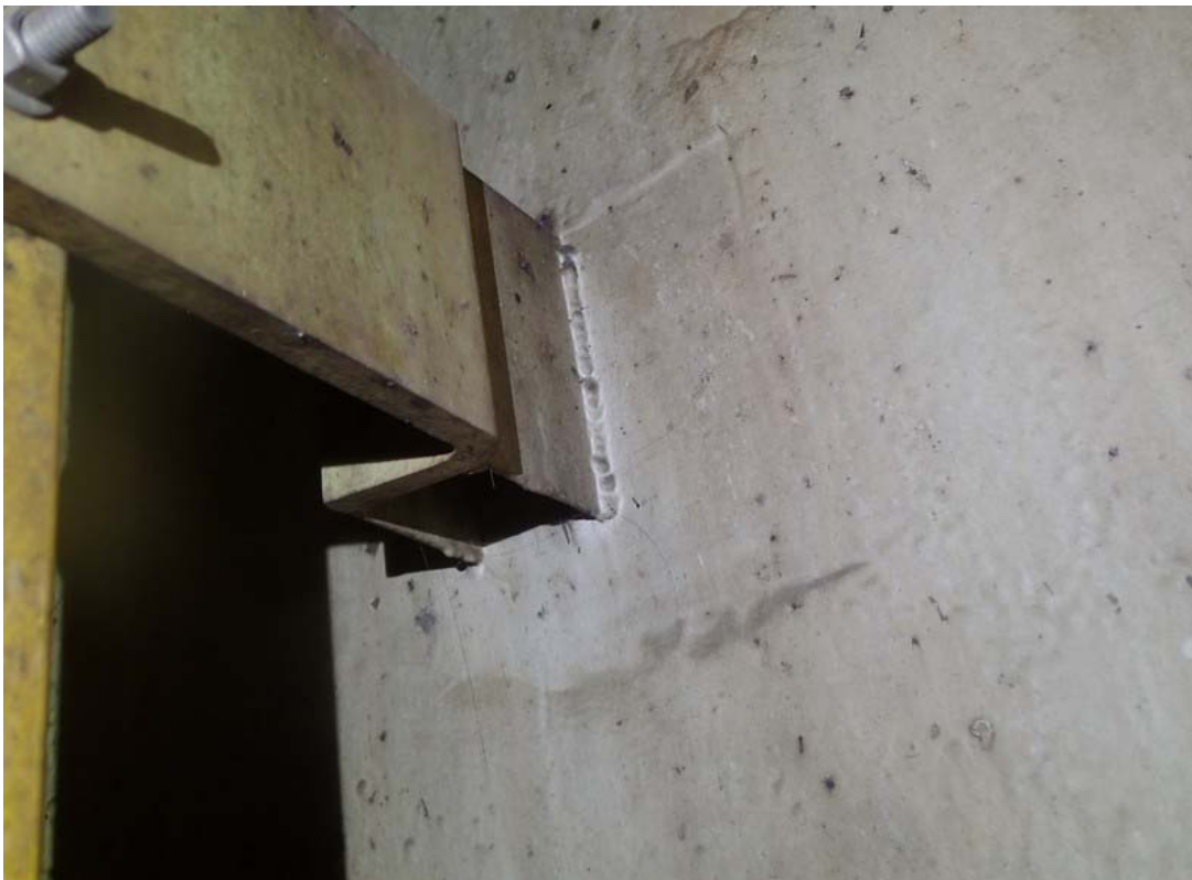
Typical ladder attachment. Ladder supports appear to be in good condition.
