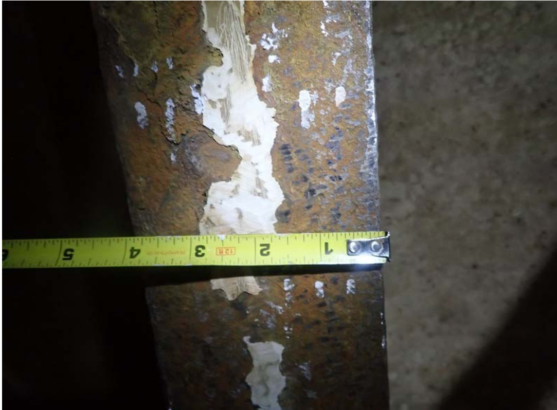
This view is taken looking upward at a sample area of a hoist beam. The bottom side of the bottom flange is shown after removal of most of the rust. The flange is approximately 4" wide.
