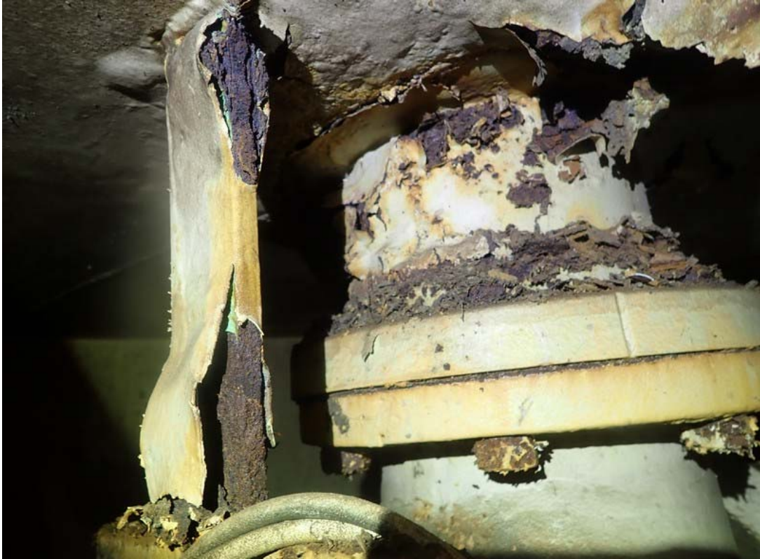
Pipe hanger on interior ceiling. Significant corrosion damage is present.
