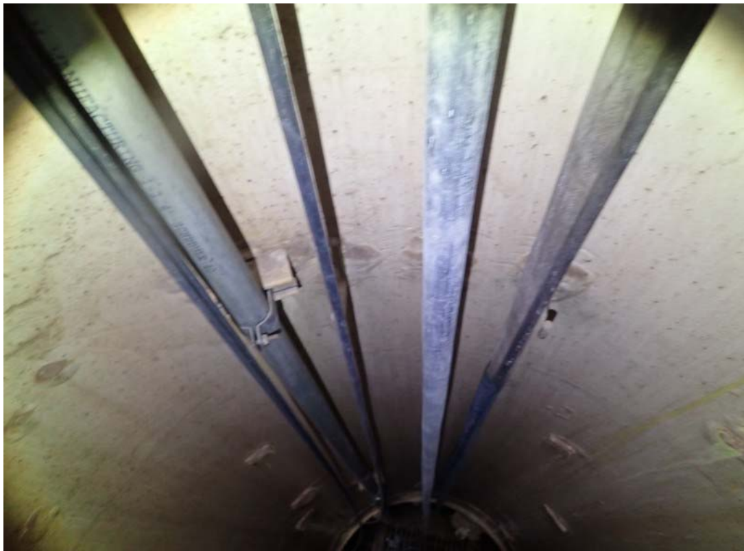
This view shows the conduit in the access tube.
