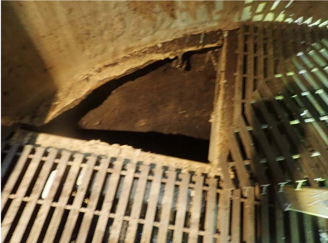
Decking pulled away to view the conditions at the perimeter flange that appears to provide some support of the grating.
