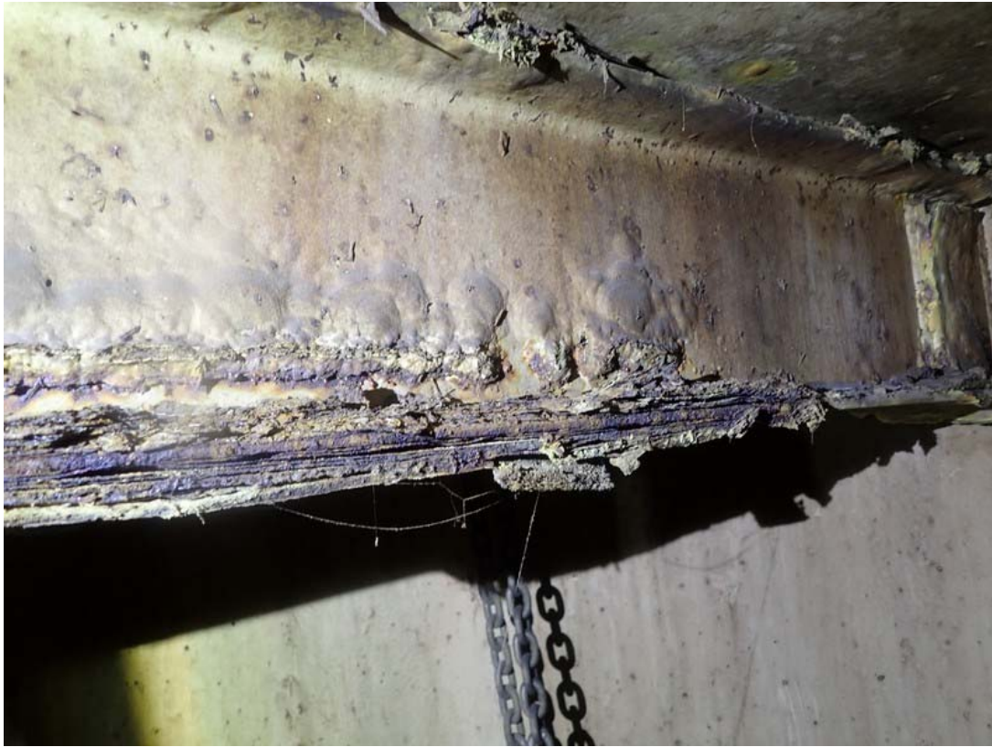
This view shows a hoist beam with what appeared to be some of the worst corrosion. This area was selected to be a sample area for rust removal, measurement and evaluation.
