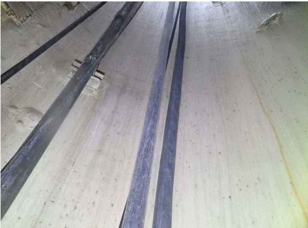
Conduit in the access tube.
