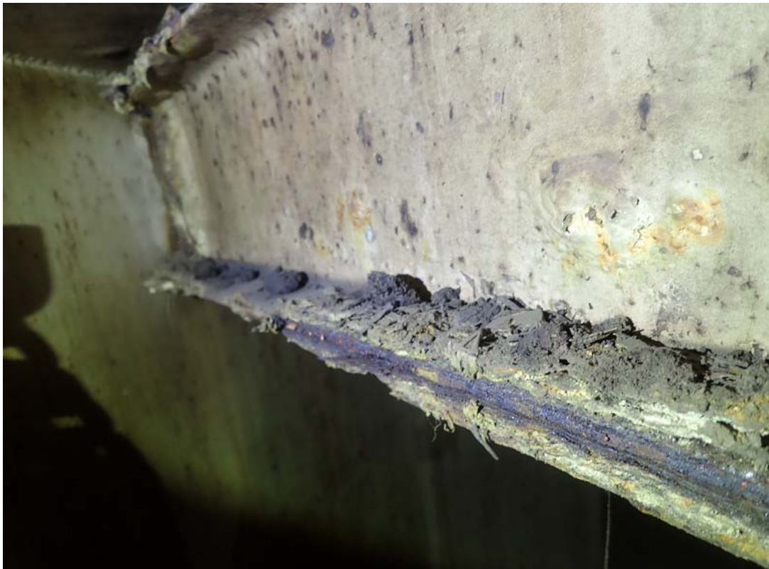
An additional view of some of the worst corrosion on the bottom flange of the hoist rails.
