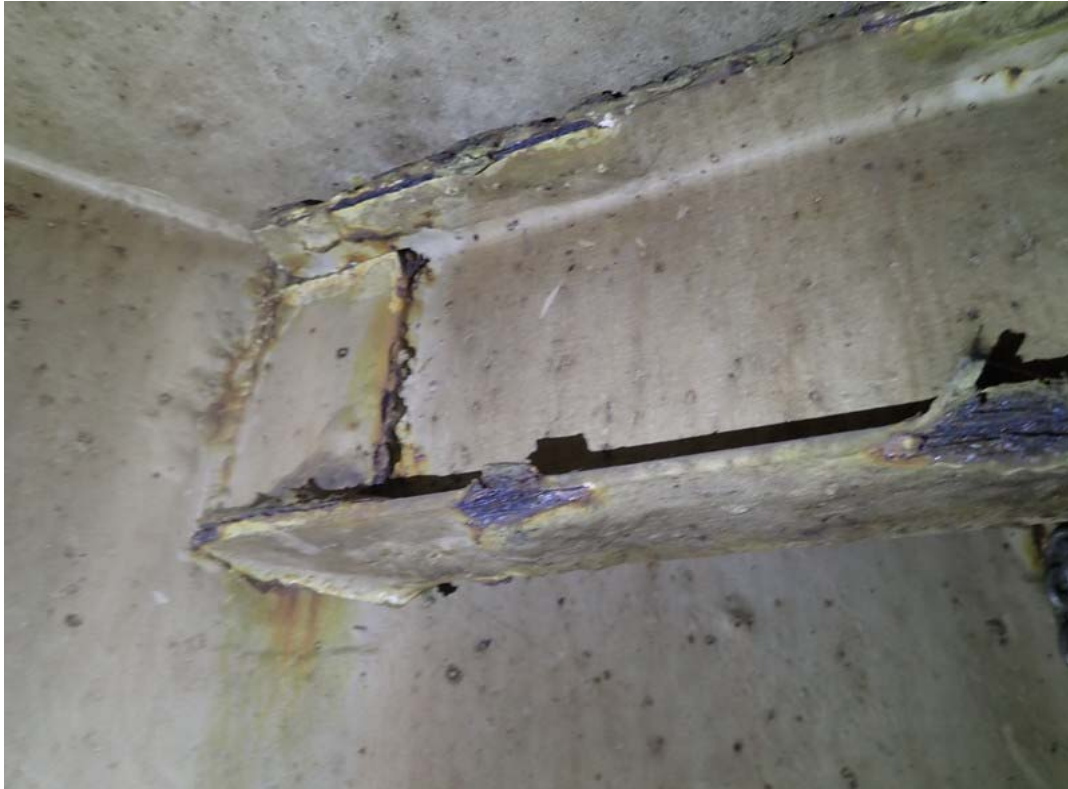
Hoist rail end connection. This view shows the typical condition of the beam rail to shell connection. The side shown is toward the center of the lift station.
