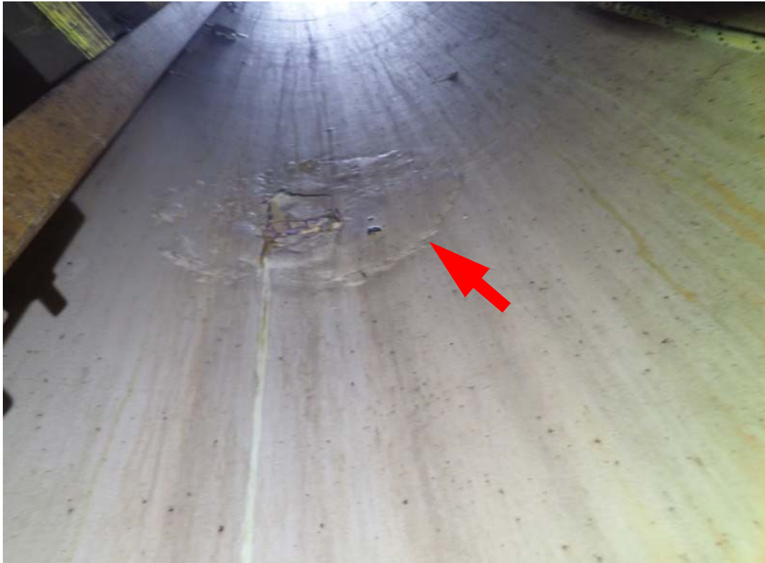
This view shows an area of the access tube. Damaged coating is visible at the arrow. Corrosion is present. under the coating.
