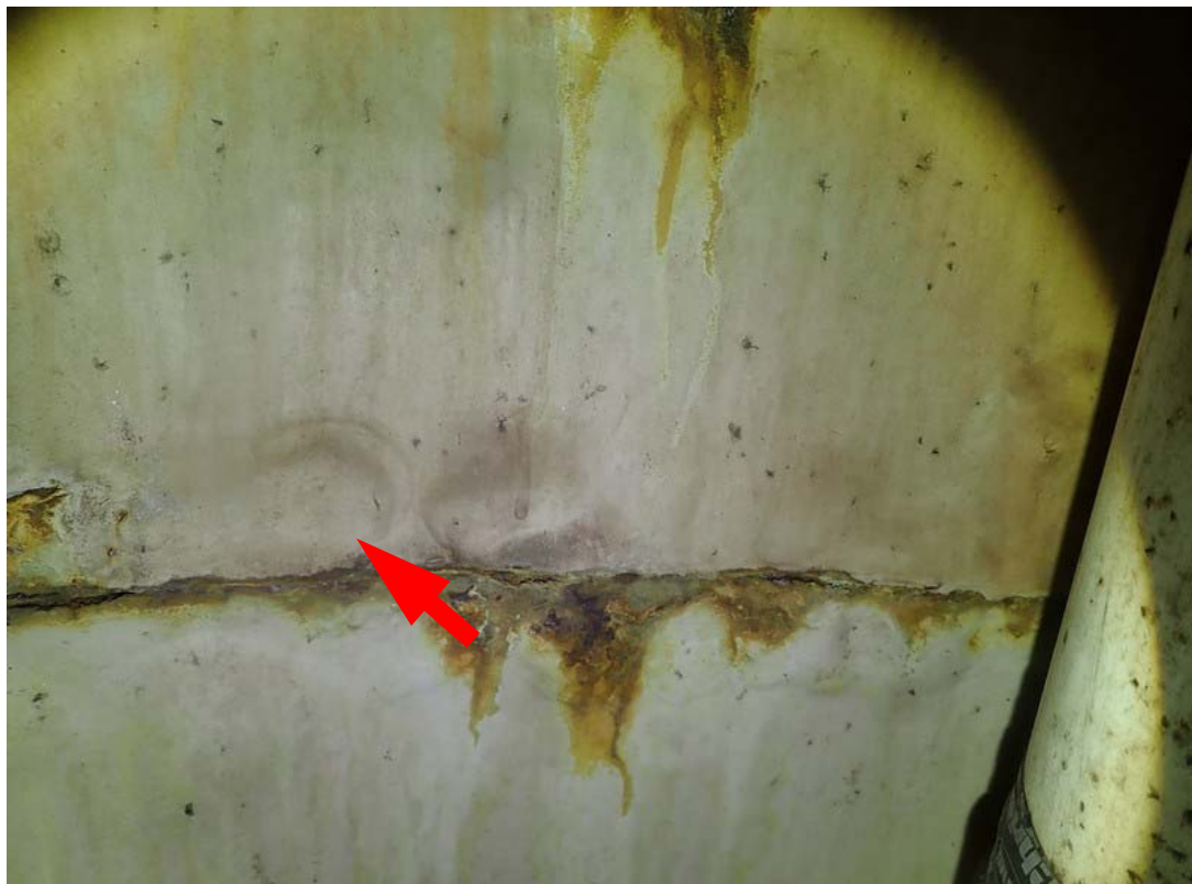
Access tube with corrosion at the joint between sections. Large blisters are visible at the arrow. The light wall PVC tube on the right appeared to be suspended only at the top.
