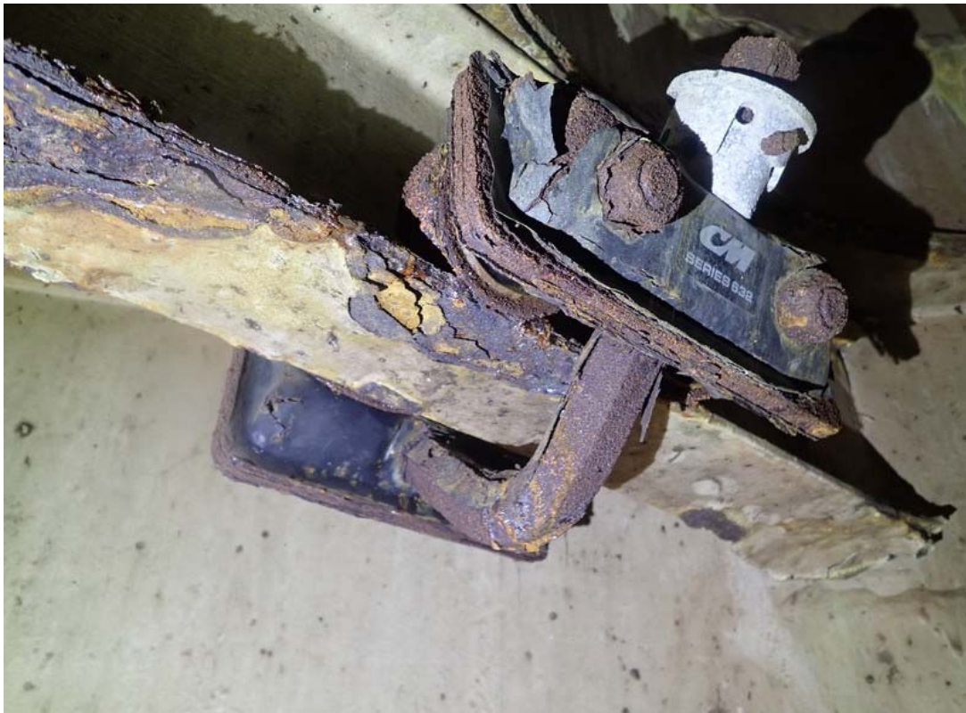
Hoist trolley in place on the northern end of the west rail. The hoist trolley is severely corroded along with the beam. It is recommended that this trolley be taken out of service immediately.
