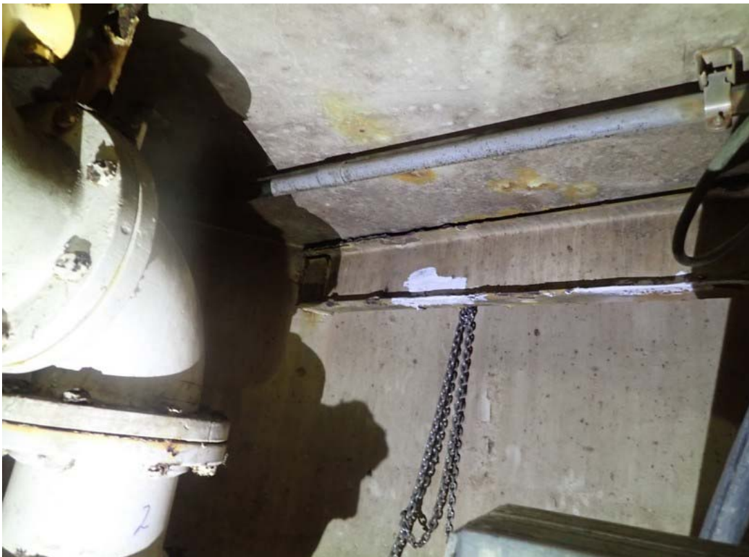
This is an additional view of coating spot application. In this photo the west rail is shown.
