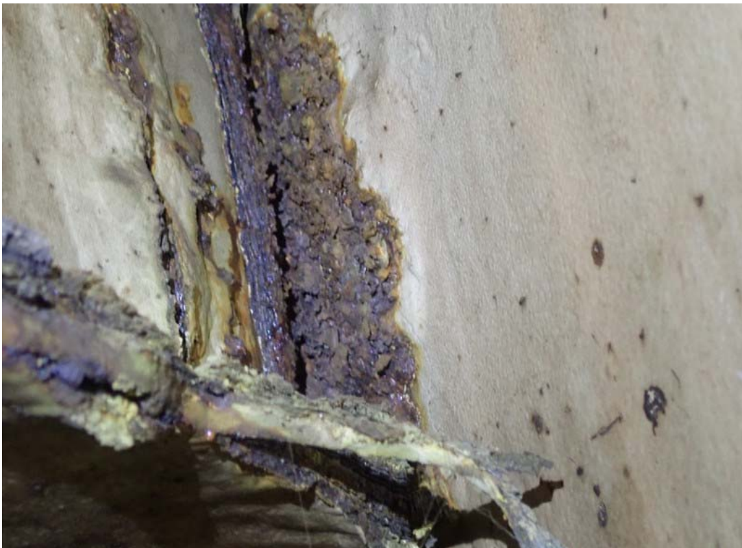
Inaccessible side of the eastern hoist rail at the shell connection. Severe corrosion is present. Measurement and evaluation of corrosion was not completed due to access restrictive geometry on the "outer" side of the attachments (shown).
