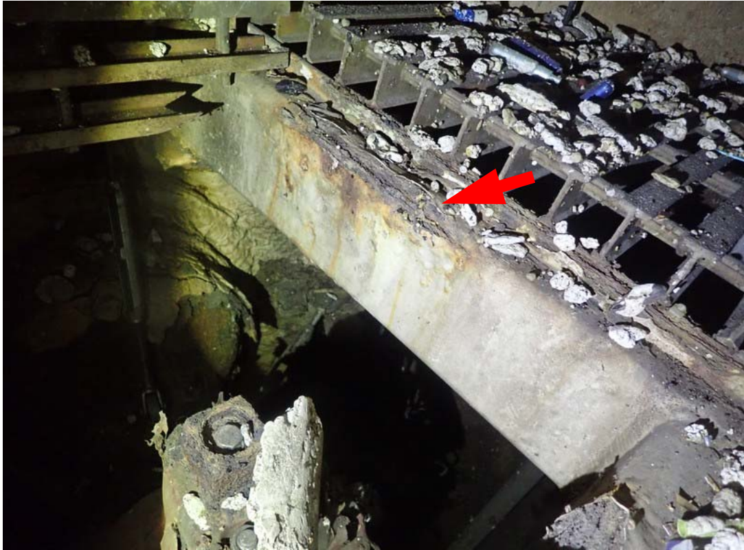
View with grating lifted to check conditions. Serious corrosion and significant metal loss are present in localized areas such as the grating support structure (arrow).
