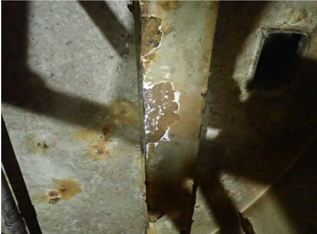
This view shows the typical sample area after most loose corrosion product was removed.
