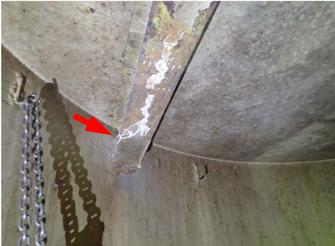
An additional view of some of the south end of the eastern beam from below. The arrow indicates the "outer" side of the hoist beam to shell connections that were inaccessible without abrasive blasting or similar cleaning methods.
