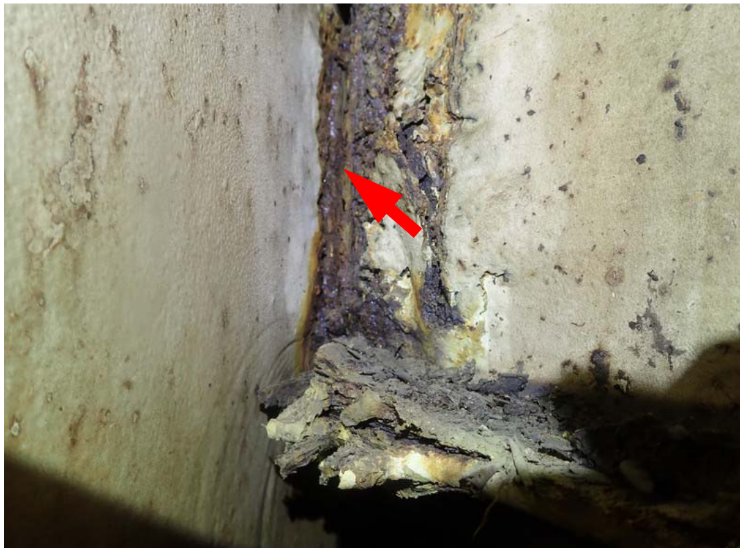
This view shows the typical condition at the hoist rail to shell connections at the outer side of the rails (opposite side as shown in the top photo). The design detail has created a crevice at the connection (arrow). The critical area is inaccessible for inspection and maintenance.
