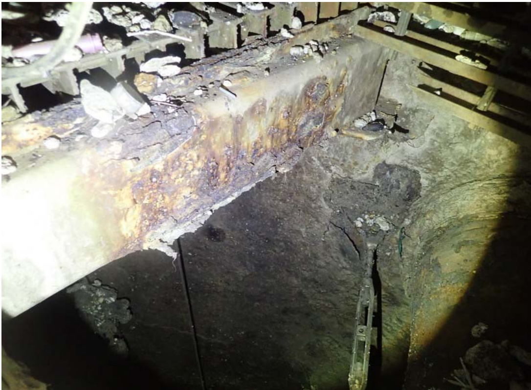
Another view of the deck support structure and pipe support turnbuckles.
