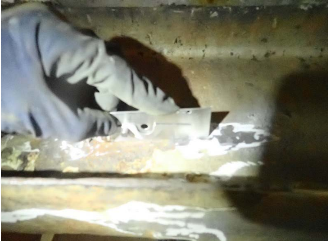
Measuring material loss on a sample area of the east hoist beam. Sound paint and metal are present adjacent to this area of localized corrosion that was checked.
