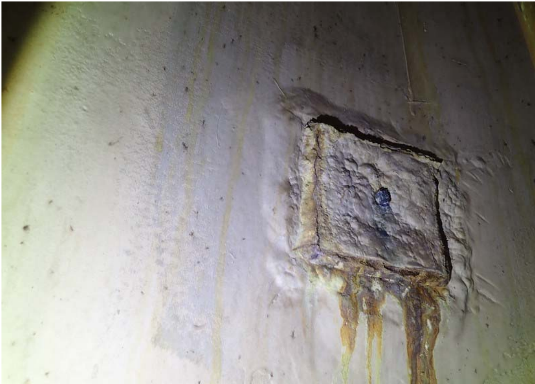
Typical corrosion at failed coatings in the access tube. Coating failures are present on most attachment point and joints in the shell of the access tube.
